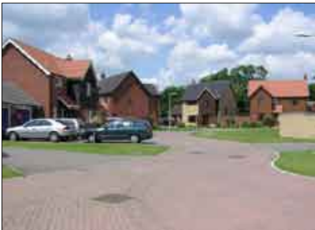
Piper’s Meadow development – spacious with clean cut lines
