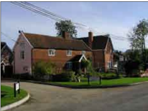
Willow Farm Cottage in 2005 - after the completion of the new housing development
