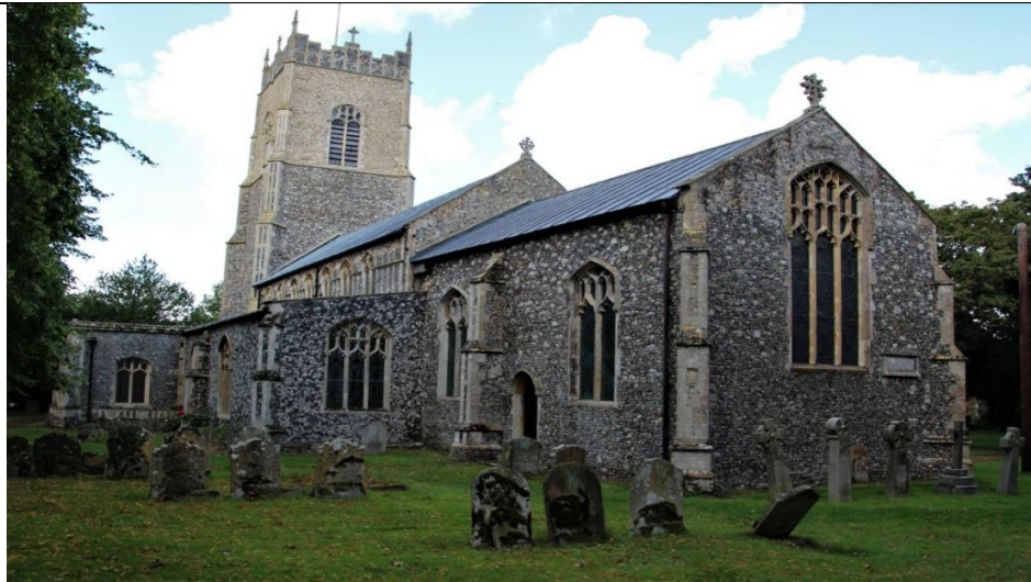
Church looking north and west (eastern elevation)
