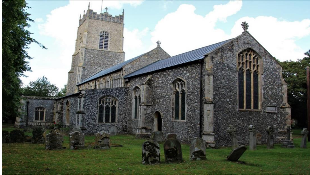
Church looking north and west (eastern elevation)
