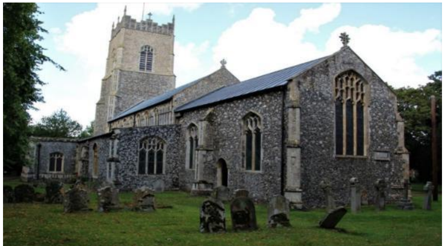
Church looking north and west (eastern elevation)
