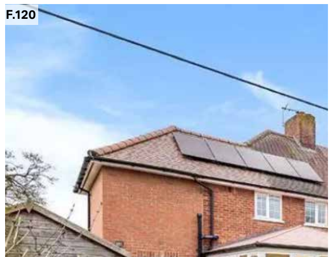
Figure 120: Solar panels installed on the south-facing pane of the roof of existing house in Wetheringsett. (Source: onthemarket.com)
