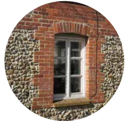
FLINT FAÇADE WITH RED BRICK WINDOW TRIM
