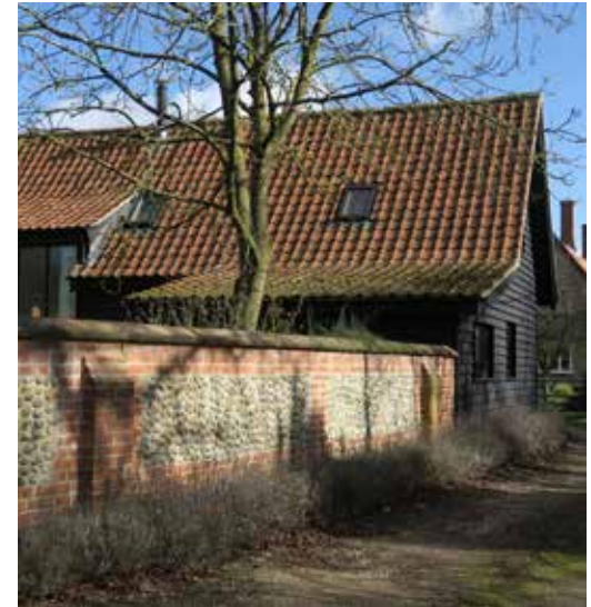
Renovated house with black weatherboarding and pantile roofing and a pebble and red brick external wall. AECOM
