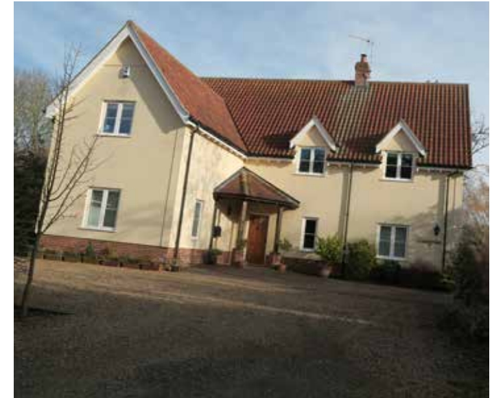
Figure 50: New house with traditional Suffolk architectural elements such as pantile roofing, high-pitched gables, and yellow render.
