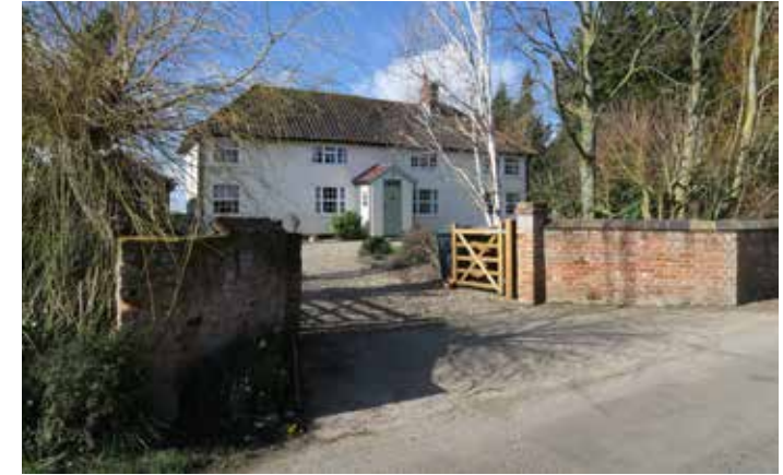
Figure 25: Brick and timber gateway framed by taller vegetation.
