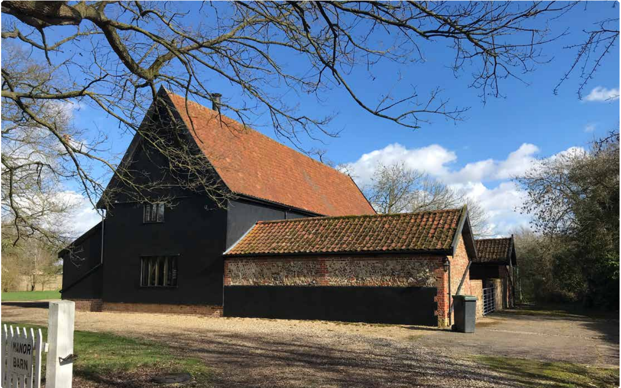
Figure 56: Grade II listed timber-framed barn with plastered and tarred façade.
