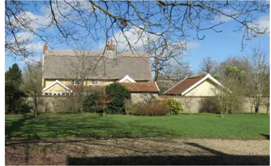
Figure 34: Small cluster showing a main building mass (thatched roof) and smaller secondary masses (pantile roofs).
