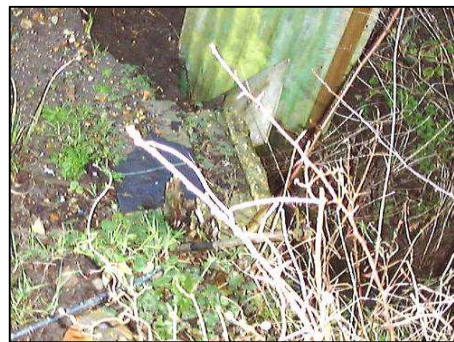
Ditches need proper maintenance. Their potential to help or hinder flooding needs to be better understood and managed
