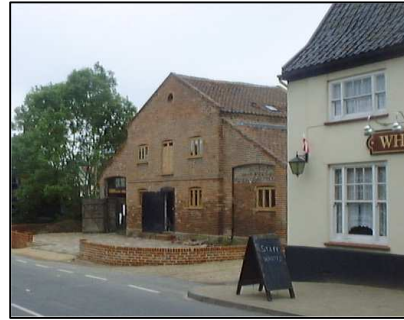
The White Hart stable block once on the "Buildings at Risk" Register being converted into a dwelling
