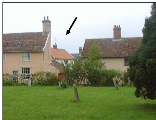
A new building within the Conservation Area seen from the churchyard, through two of the village's oldest buildings. It replaced a semi derelict garage and fronts onto Queen Street. The use of modern, bright orange concrete roof tiles mars an otherwise reasonable solution for the site.
