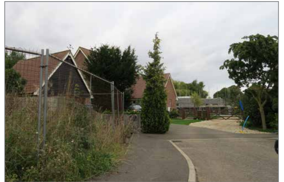
Fig. 1.9 View of Site 6 looking north from Meadow Way
