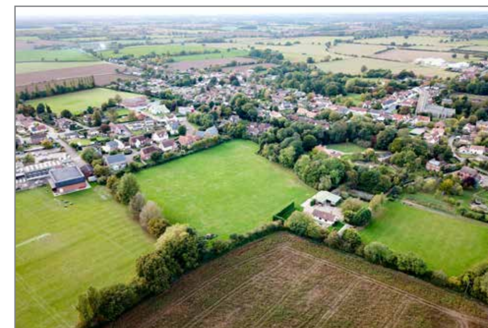
Fig. 4.3.3 Aerial view of Site 2
