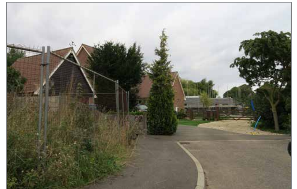
Fig. 3.7. View of the proposed site access from Meadow Way
