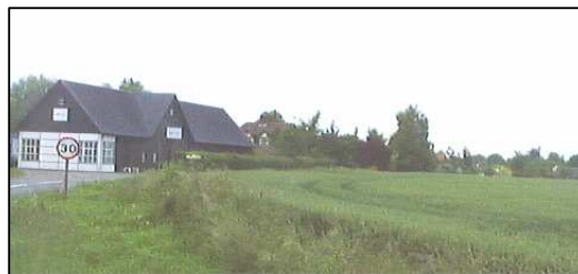
Like them or dislike them, these light industrial units are a good attempt to fit something into the landscape. They in turn sit reasonably well with the older buildings on the north side of New Street
