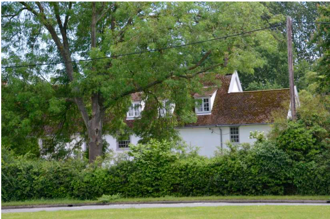
Grade II listed building on Church Road
