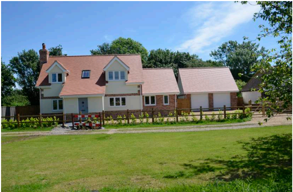
New build on the Green
