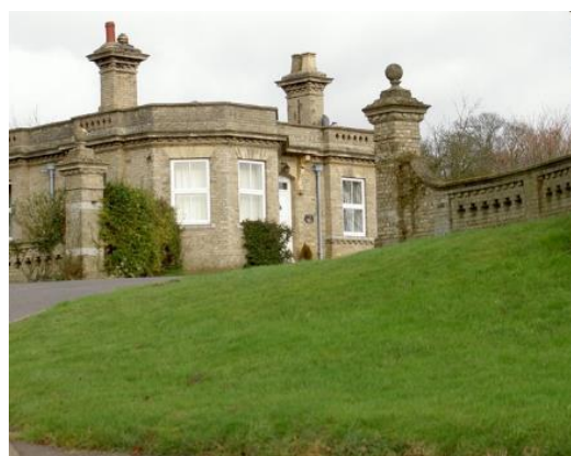
Redgrave Hall Lodge, Hall Lane
