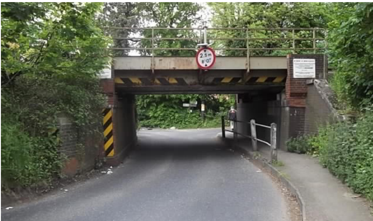
Coddendam Road Railway Bridge
