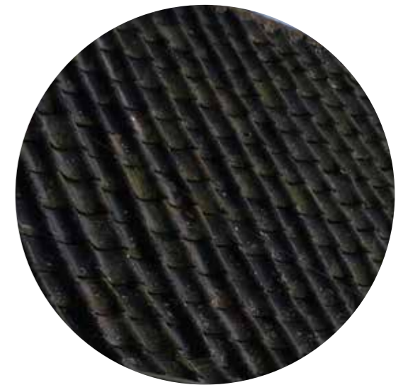
CLAY PANTILE ROOF
