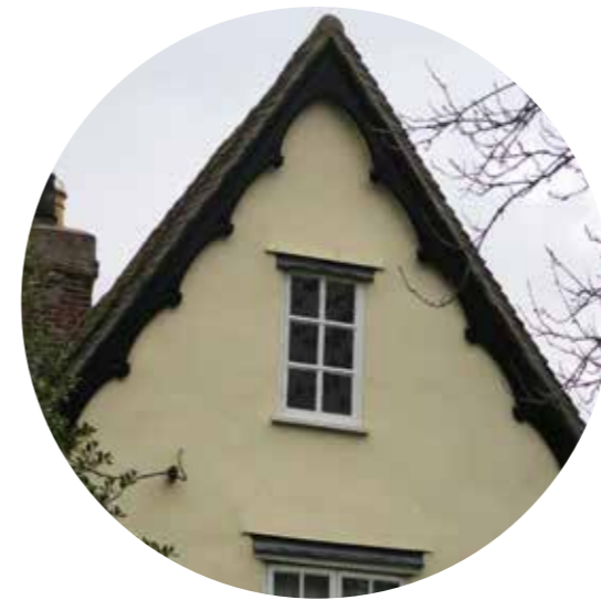
DECORATIVE BARGE BOARD
