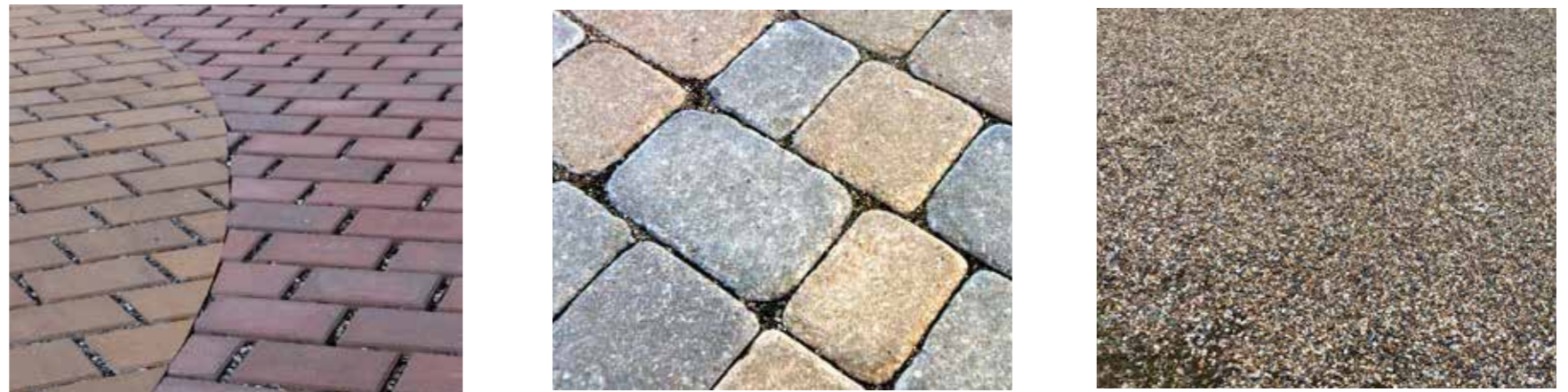
Figure 64: Examples of permeable paving treatments: clay pavers, stone/precast concrete setts, and unbound gravel.
