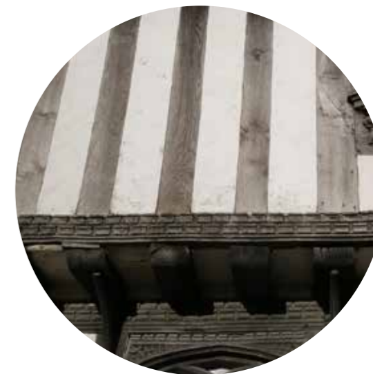
EXPOSED TIMBER FRAMING
