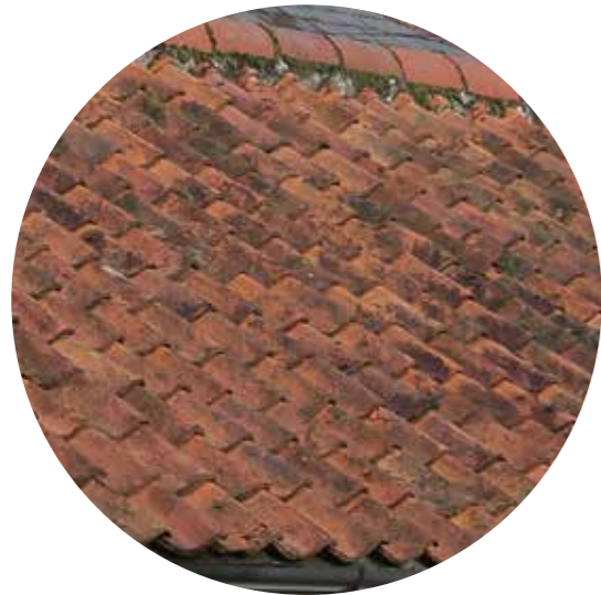
CLAY PANTILE ROOF
