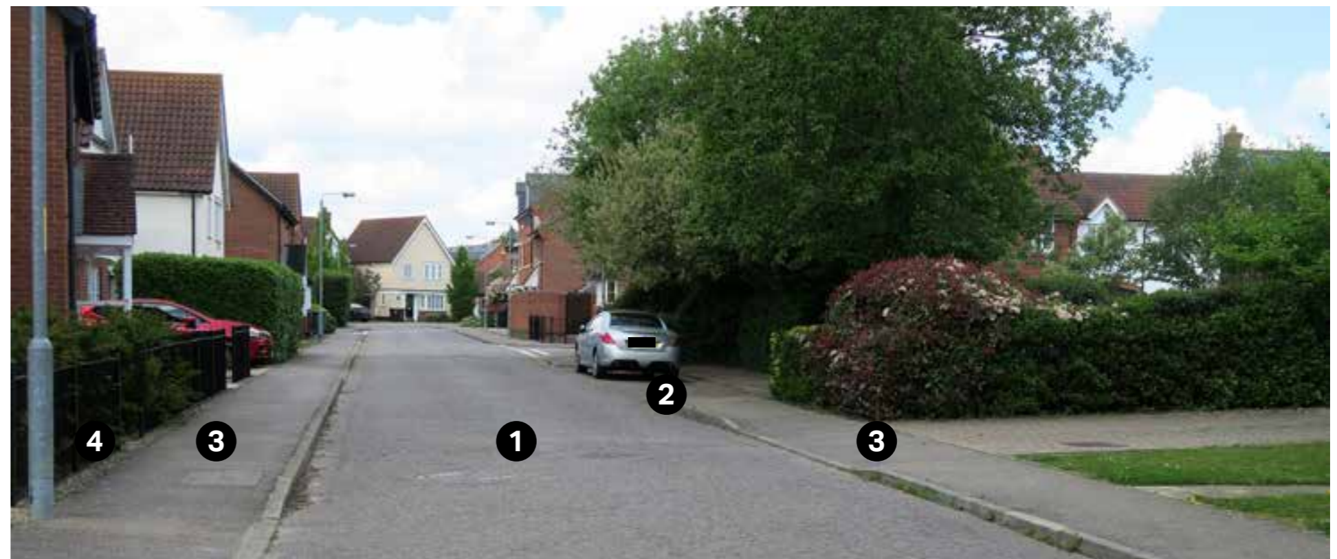
Figure 25: An example showing tertiary road framed with footpath on both sides.
