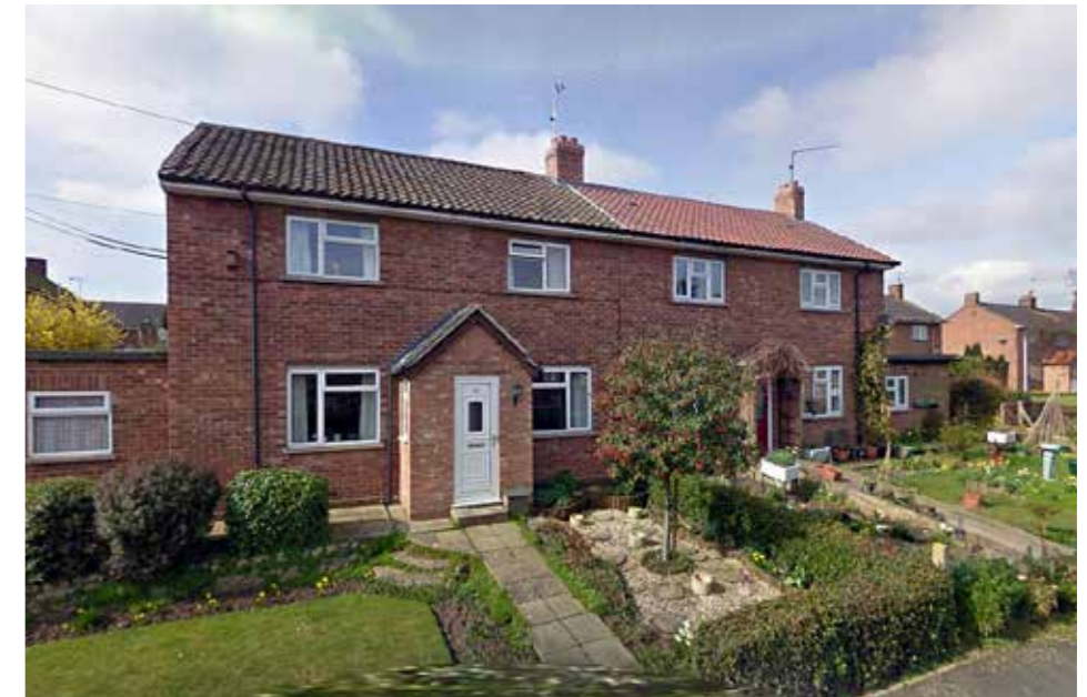
Figure 13: Semi-detached house, Crowley Road.
