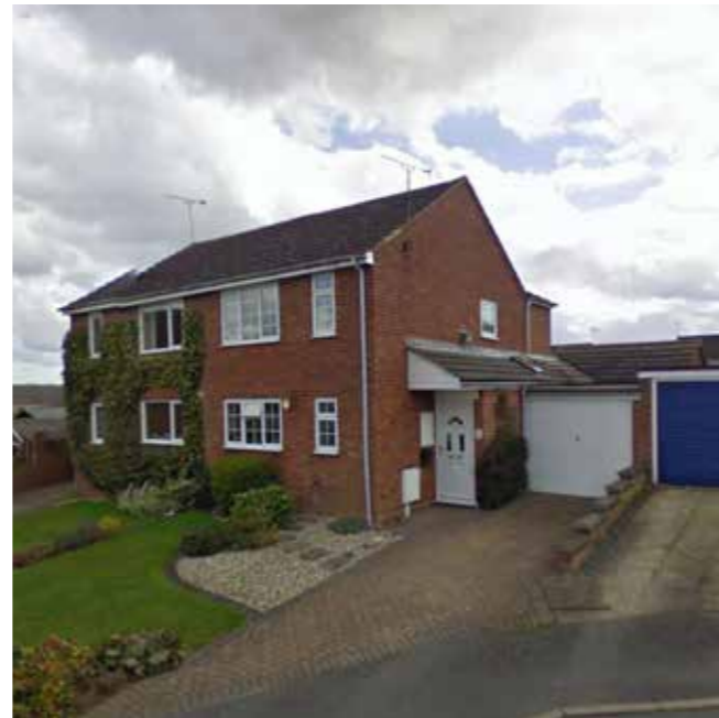
Figure 47: Gabled roof on Chainhouse Road.
