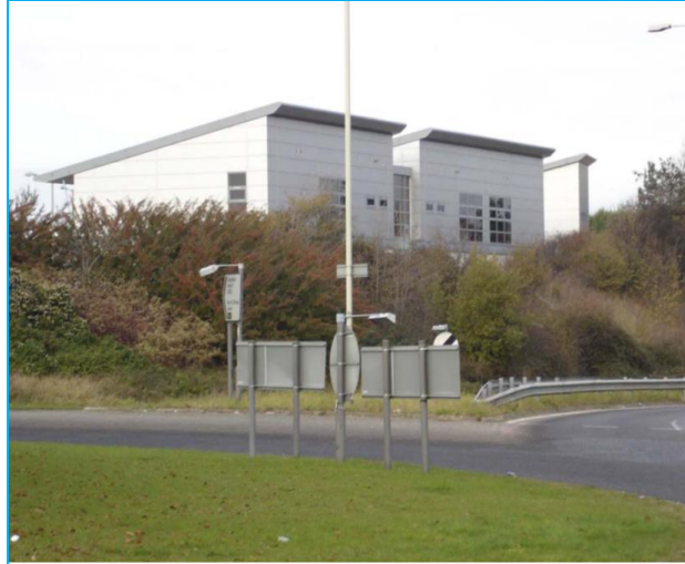
Ridge Line Offices fronting site access roundabout
