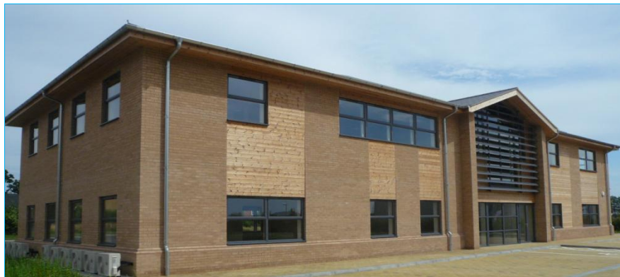
Example of office building with solar shading and light buff brickwork
