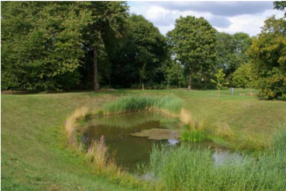
Surface water attenuation balancing pond
