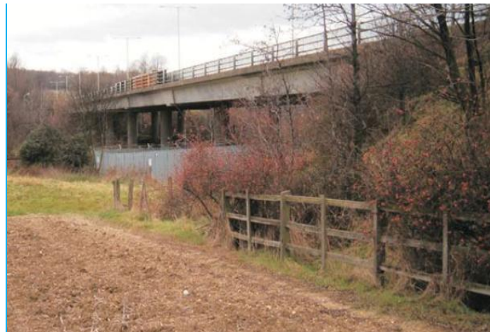
A1120 Road Embankment and Flyover at Site South Western Corner
