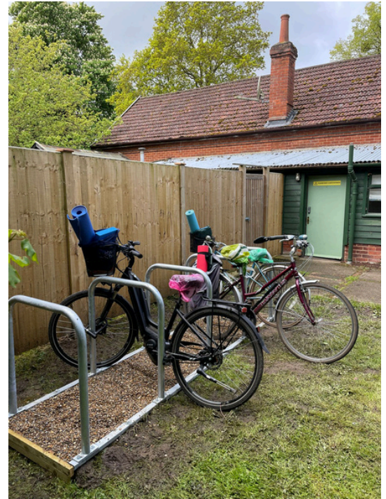
Installation of a new bike rack outside Thornhams Parish Hall
