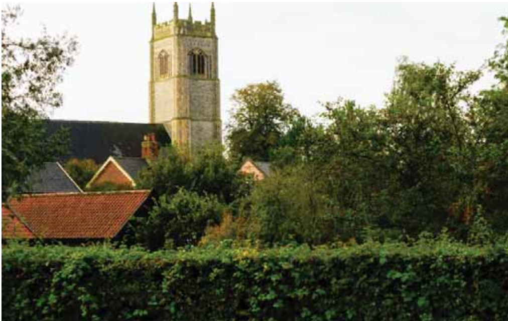
View of the Church from Gorams Mill Lane
