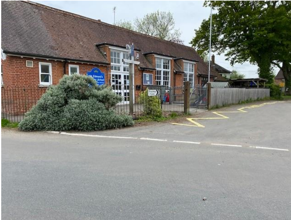
Photograph showing junction from Cross Street to Denham Low Road adjacent to school
