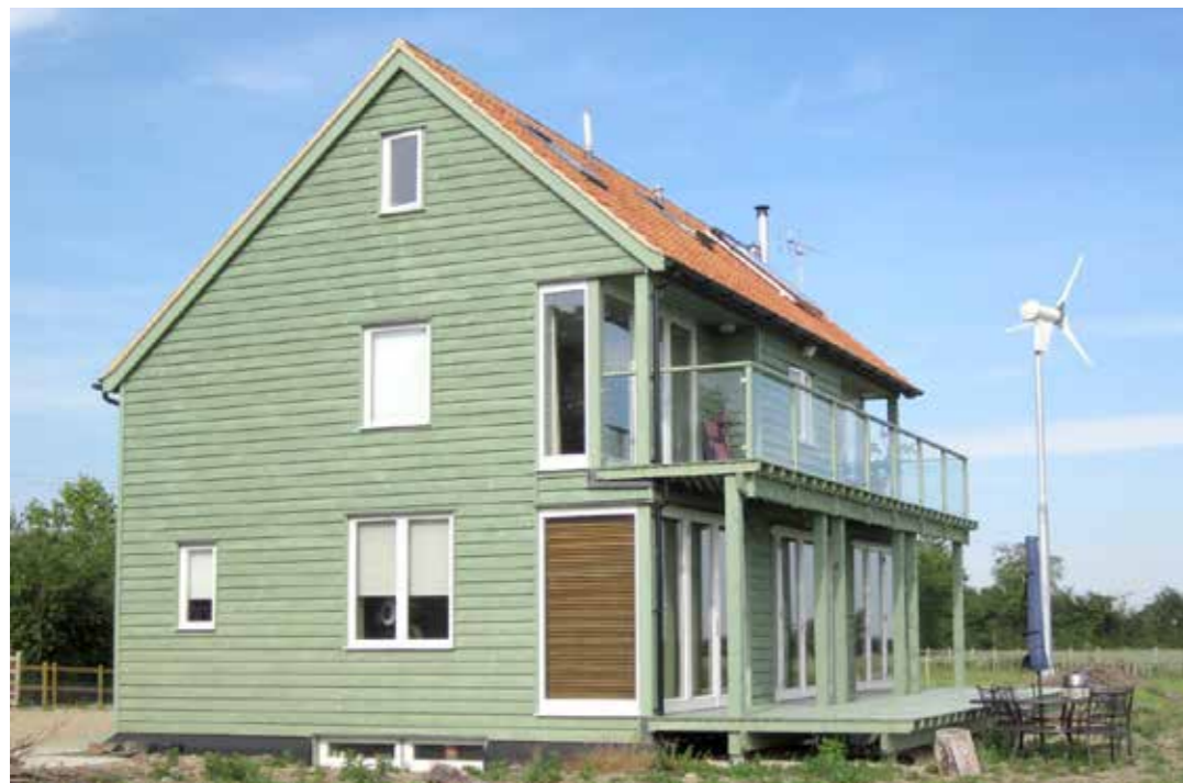
Fig 4.56. Example of contemporary architecture in Birdbrook. Sustainable house constructed to Passivhaus standards. Designed to be self-sufficient with a wind turbine, rainwater collection, reed-beds for sewage treatment and natural ventilation. RIBA East Building of the Year 2011. Photo courtesy of Modece. Source: http://www.modece.com
