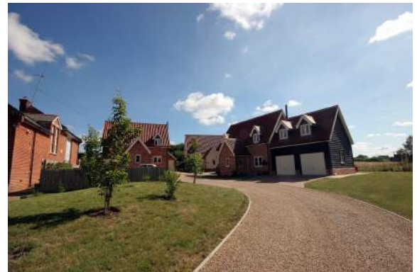
*24 Housing Scheme on former Old School site, Cratfield Road
