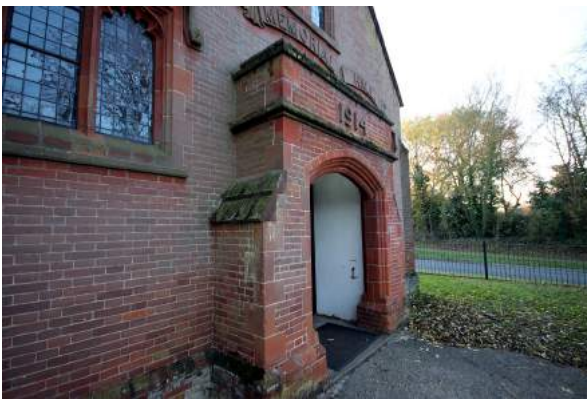
*7 Terracotta detail around porch entrance, Sancroft Hall
