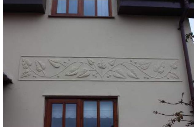
*4 Close up of pargetting on house – Victoria Terrace
