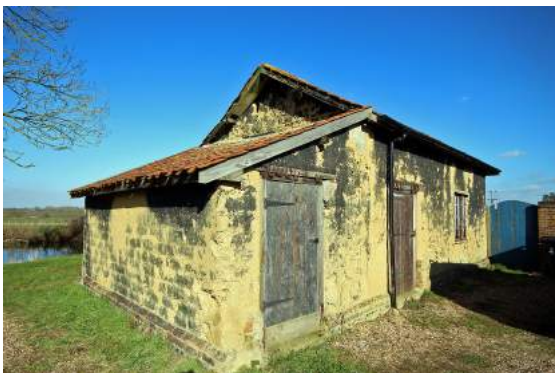
*9 Clay lump stable and small barn
