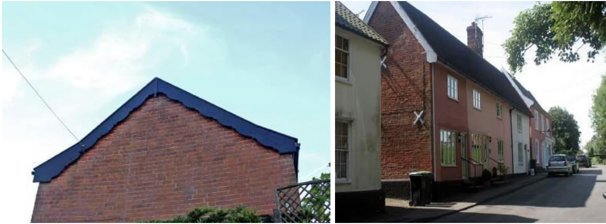
Rooves – barge-boarding and overhanging eaves
