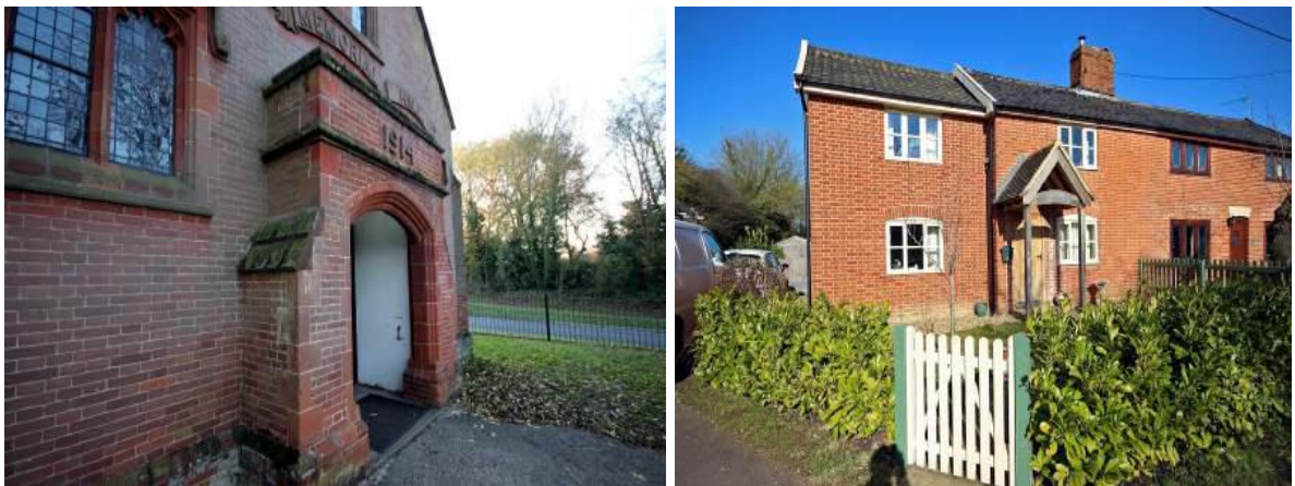
Details – porch details and brick arches
