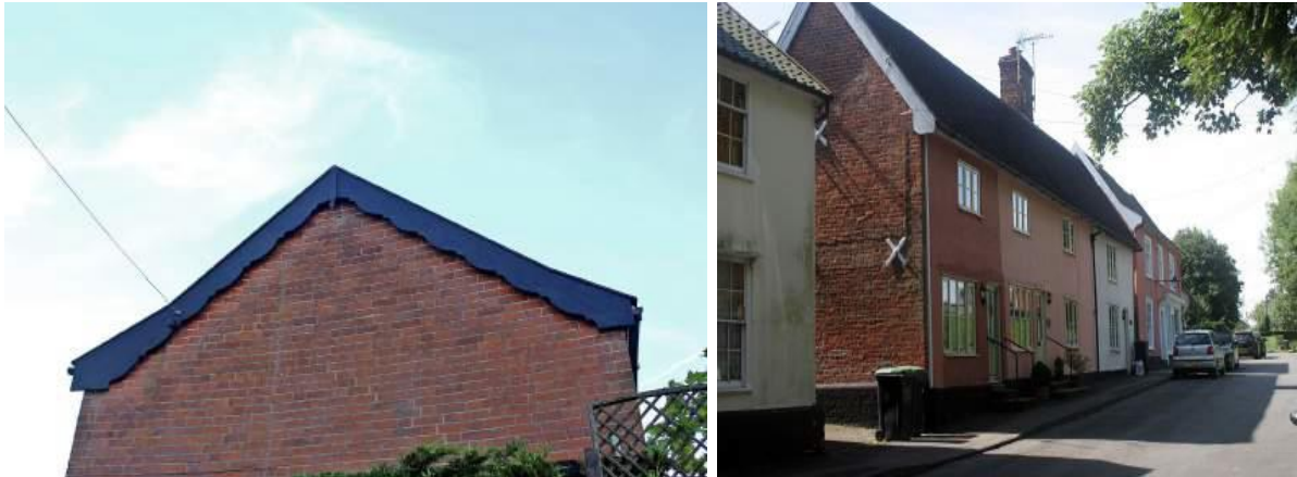
Rooves – barge-boarding and overhanging eaves
