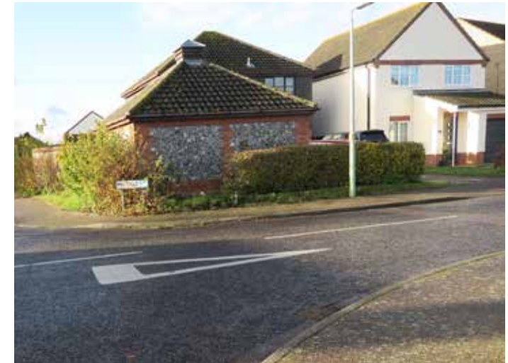
Building with traditional brick trim and flint infill forming a gateway to the post-war Millfield development
