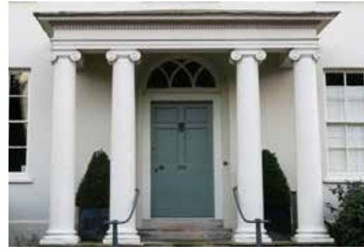
Projecting porch with Ionic columns
