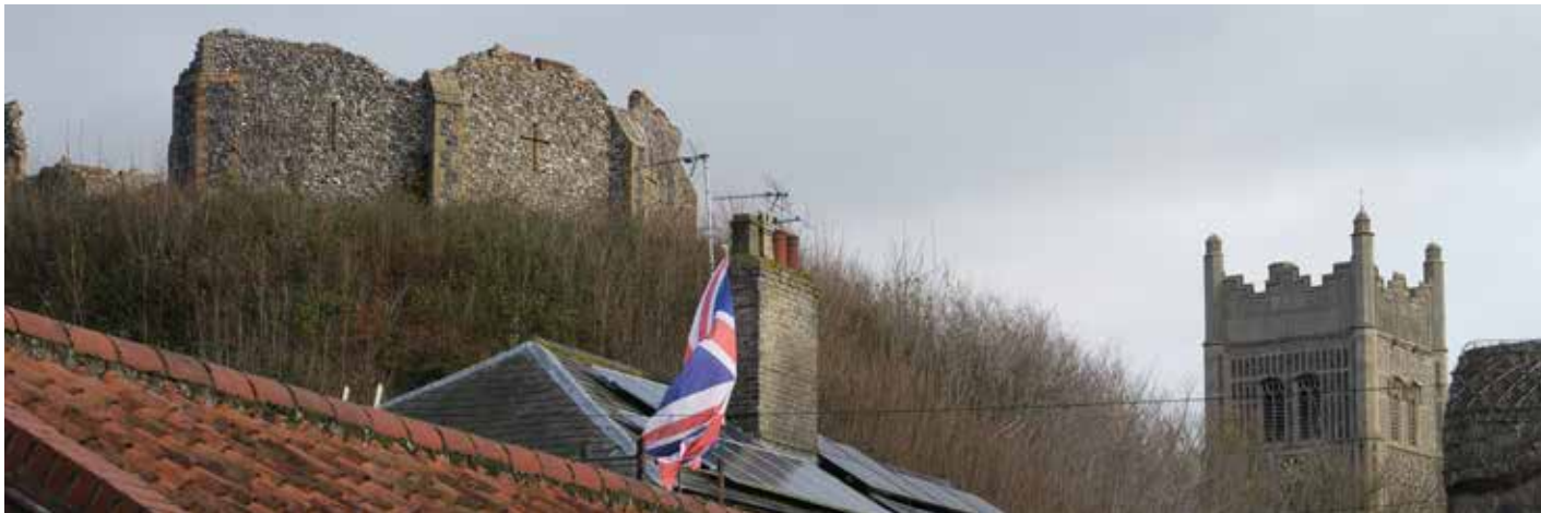
View towards Grade I listed Eye Castle and the Church of St Peter & St Paul
