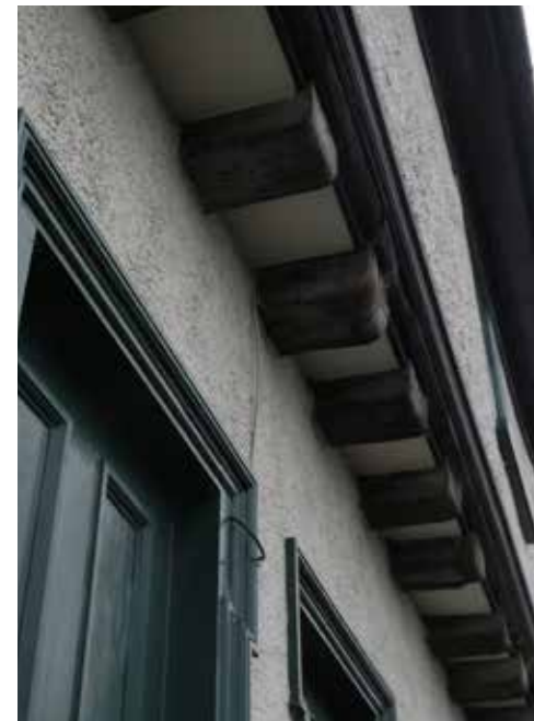
Jettying upper storey with exposed wooden beams
