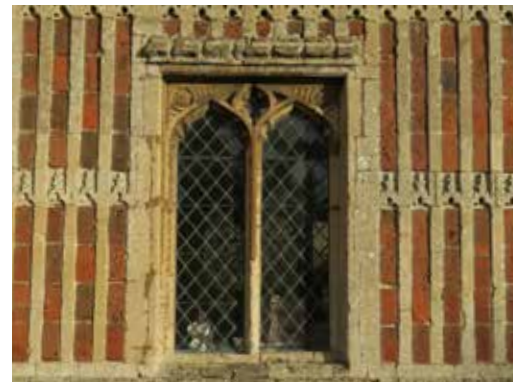
Gothic window with red brick and stone banding
