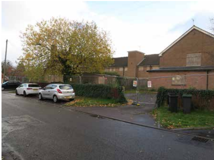
Back of Paddock House showing inset parking bays along Wellington Road.
