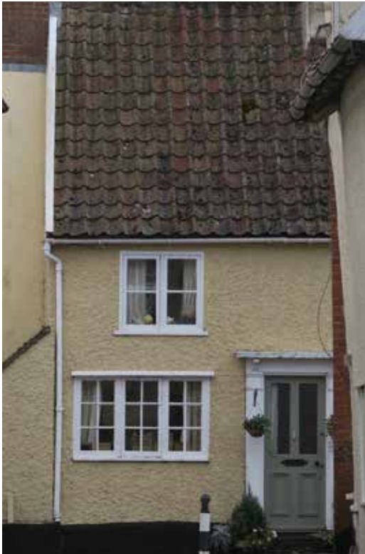
Building façade details with clay pantile roof
