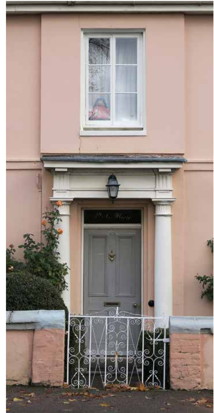
Grade II listed Bridge House
