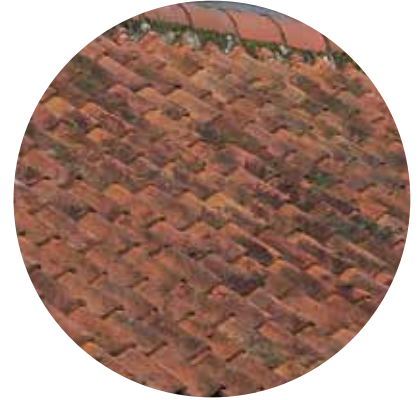
Clay pantile roof
