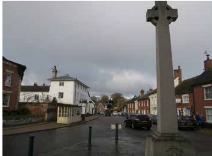
Gradual building line recesses on Broad Street create informal public squares that constitute memorable focal points and highlight local landmarks such as the Eye War Memorial in front of the Town Hall
