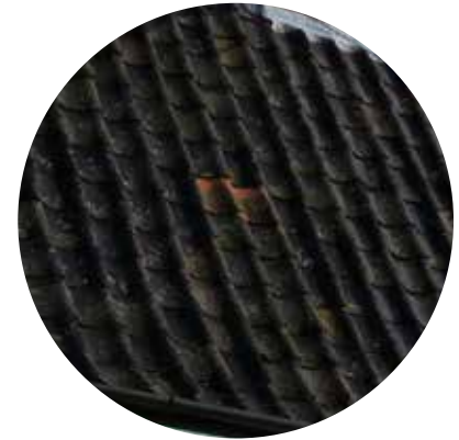
Black glazed pantile roof
