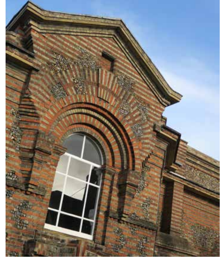
19th century Grade II* listed Eye Town Hall. Banded red and Gault brick with flint detailing of diamond and half-diamond lozenges
