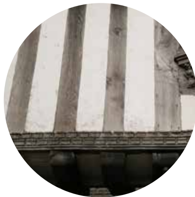
Exposed timber framing
