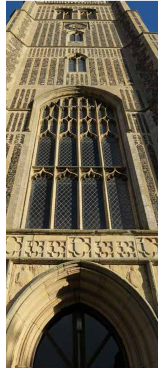
Church tower and window tracery details
