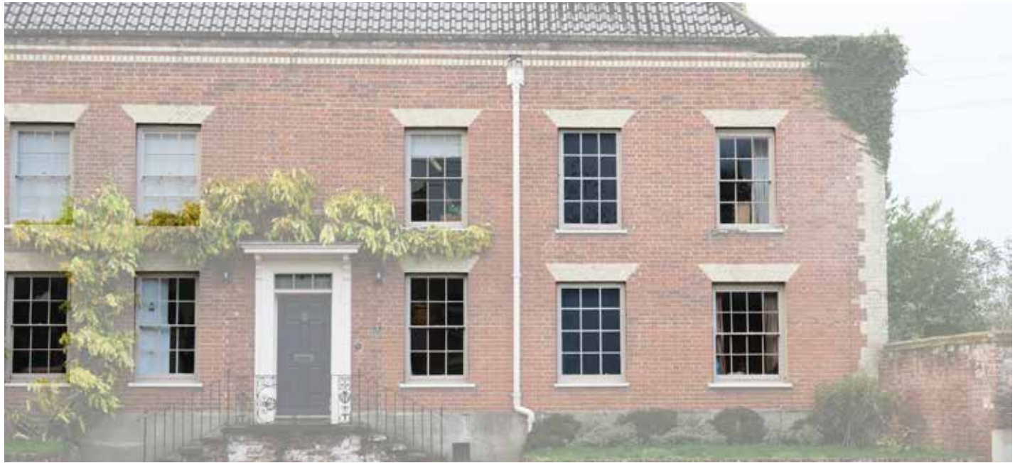
Front elevation using a formal arrangement of sash windows placed at regular intervals
