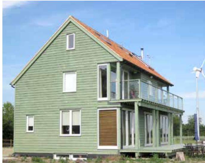
Example of contemporary architecture in Birdbrook. Sustainable house constructed to Passivhaus standards. Designed to be self-sufficient with a wind turbine, rainwater collection, reed-beds for sewage treatment and natural ventilation. RIBA East Building of the Year 2011. (photo courtesy of Modece; source: http://www.modece.com )
