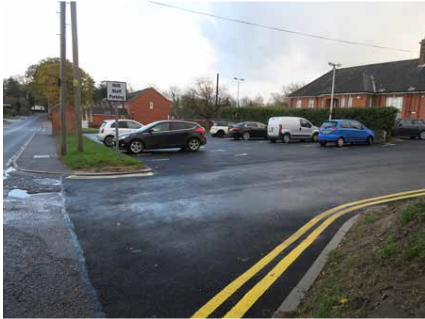
Site edge with Castleton Way showing the police station and the NHS car park
