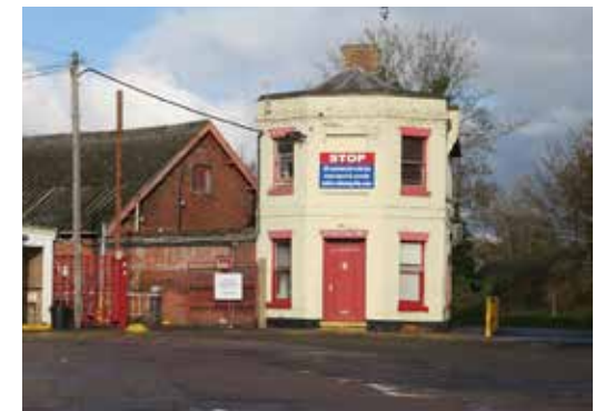
Railway station structure to be retained as part of the development
