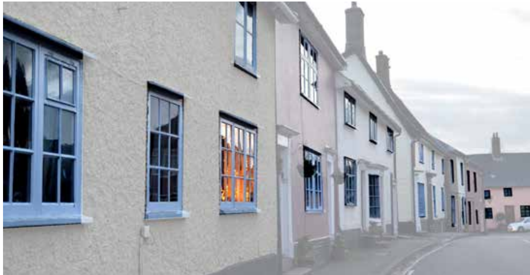
A succession of ground floor windows enables better surveillance of the public realm than long stretches of windowless walls
