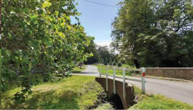
Bridge over River Black Bourn
