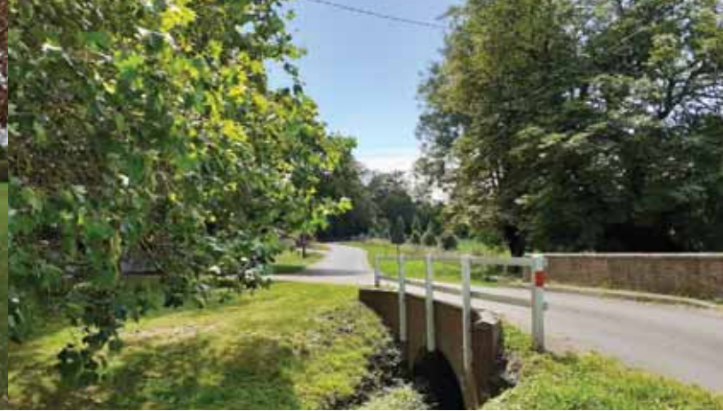
Bridge over River Black Bourn
