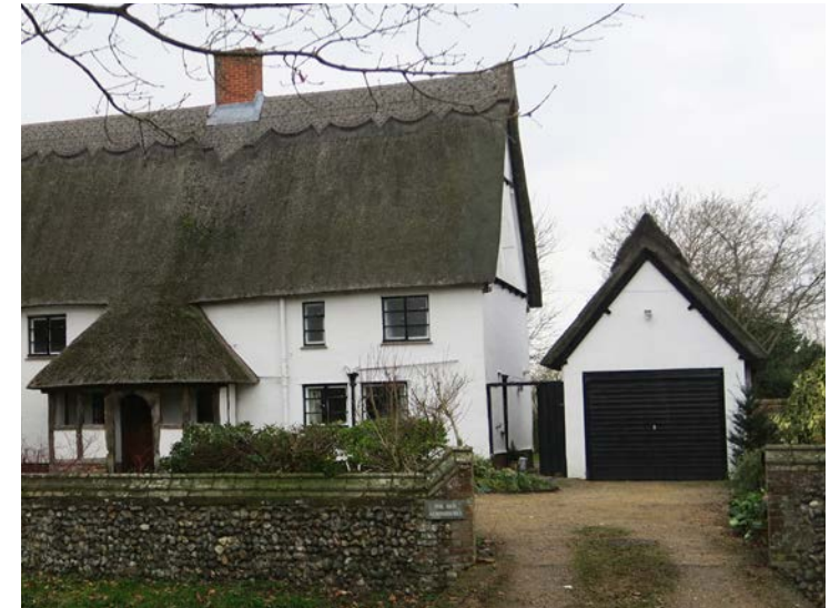
Figure 44: Side garage building with high quality finish.
