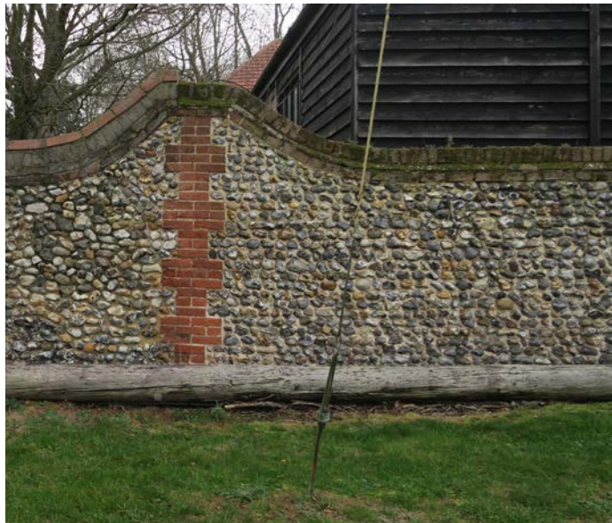
Flint wall with red brick cap and trim.
