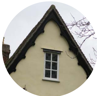
DECORATIVE BARGE BOARD
