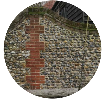
FLINT WALL WITH RED BRICK TRIM AND CAP
