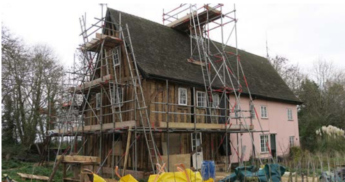
Figure 3: Grade II listed timber-framed cottage on Cross Street under restoration. AECOM
