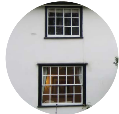
PAINTED SQUARE WINDOW FRAMES
