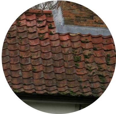
CLAY PANTILE ROOF
