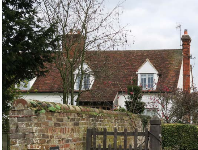
Gabled dormers on clay plain tile roof (back) and brick wall (front)
