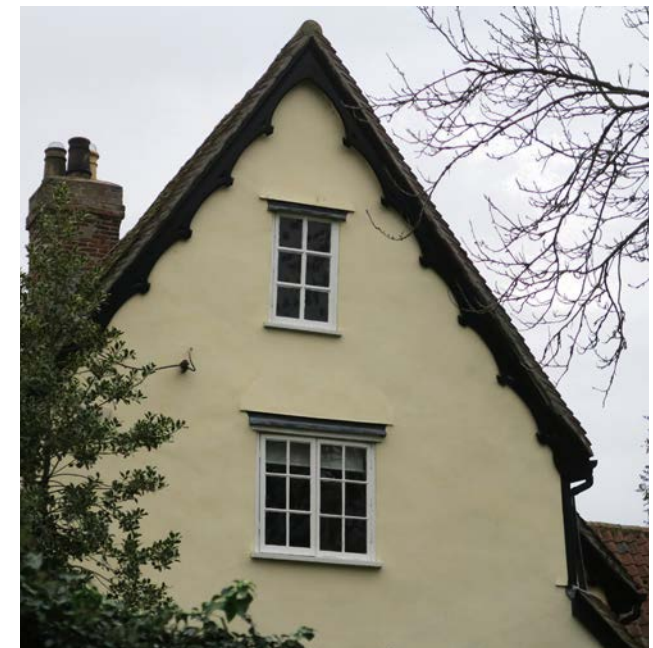
Gable with decorative barge board and rendered off-white walls.
