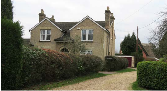
Figure 12: "Woolpit white" brick house.
