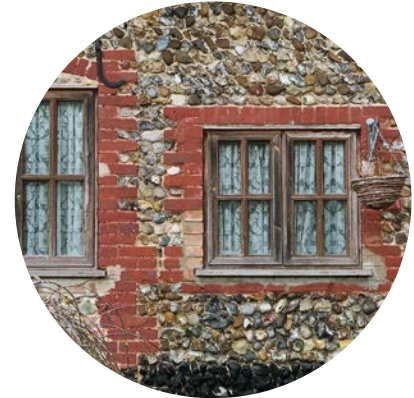
FLINT FAÇADE WITH RED BRICK WINDOW TRIM
