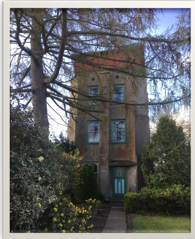
Heritage image NDHA 18 Roydon Tower House, High Road. Map location TM10174 80186
