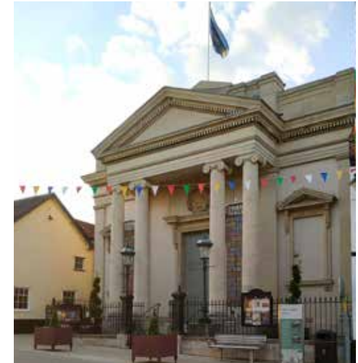
Figure 28: The Corn Hall on St Nicholas Street.
