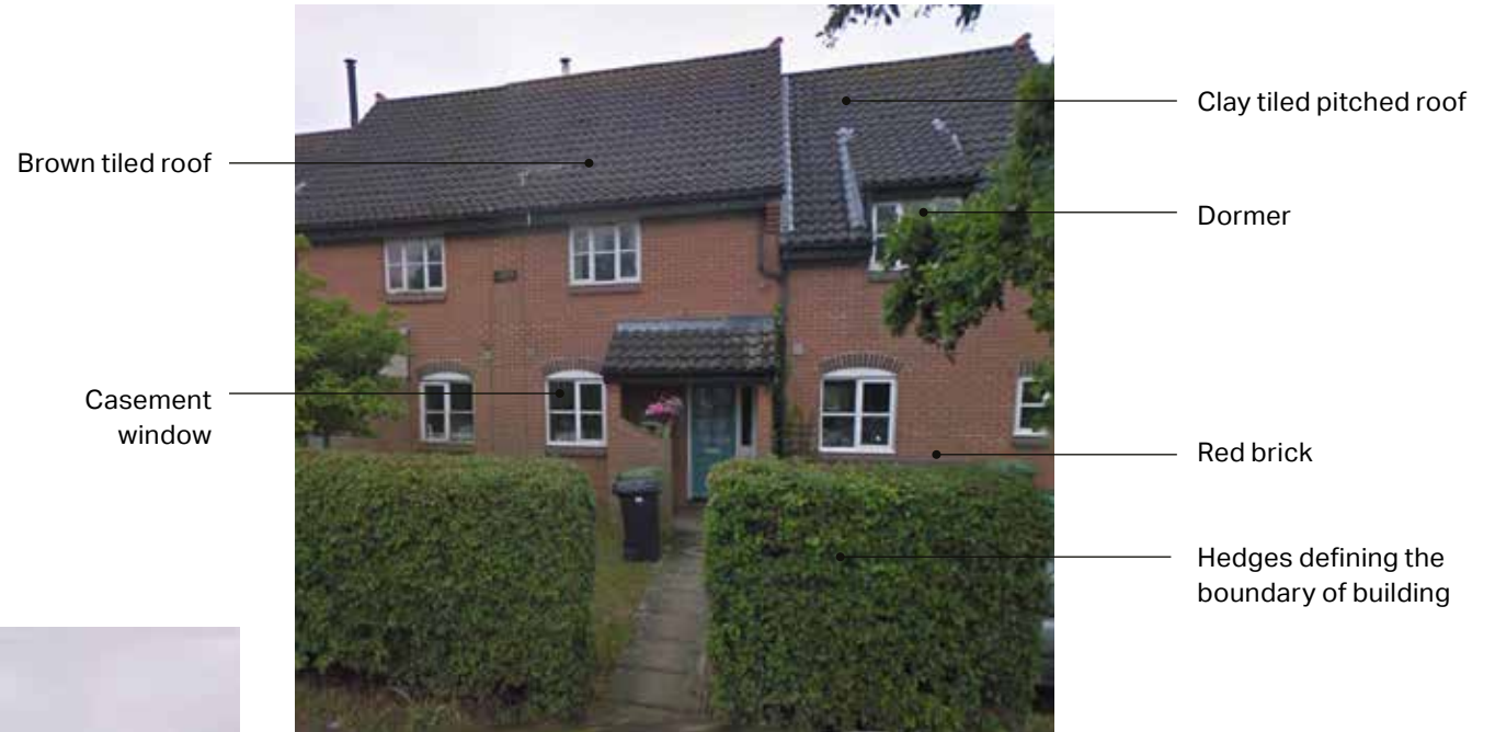
Figure 110: Red-brick dwelling with a clay tile roof on Mill Road, Burston.
