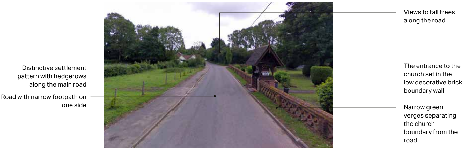
Figure 138: Street layout details along Rectory Road.
