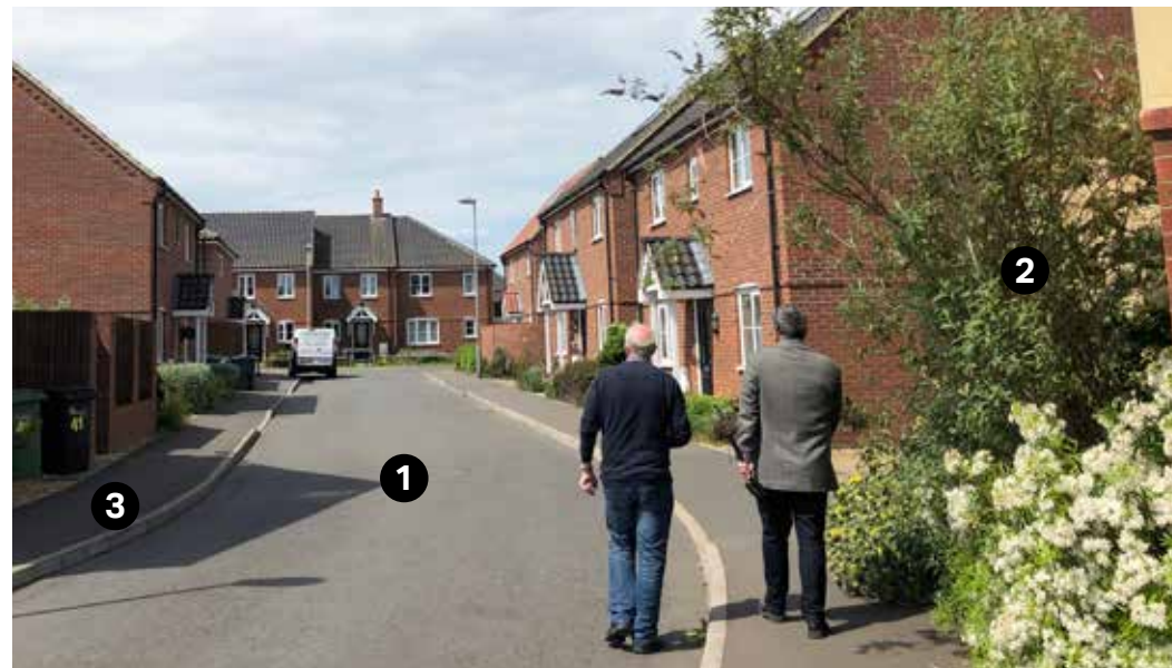
Figure 51: Tertiary road framed with footpath in both side.
