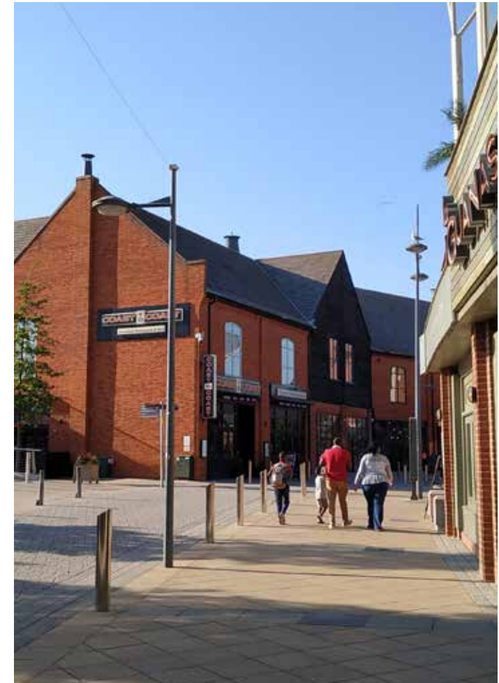
Figure 156: Example of lighting columns set at heights and positions to provide light to both pedestrian areas and the carriageway. It is recommended that LED lighting is used due to higher energy efficiency and power cost savings.
