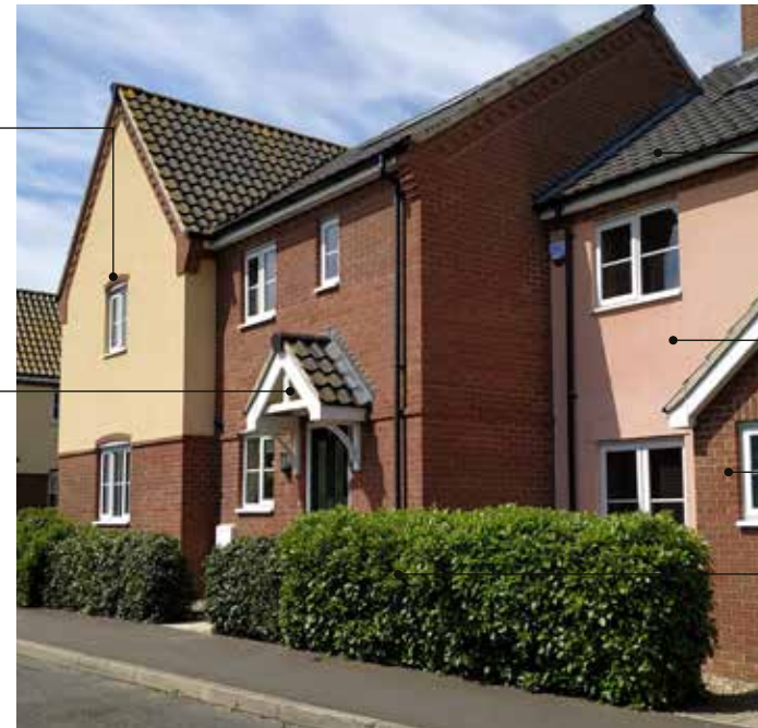
Figure 97: Building located on Spencer Crescent.
