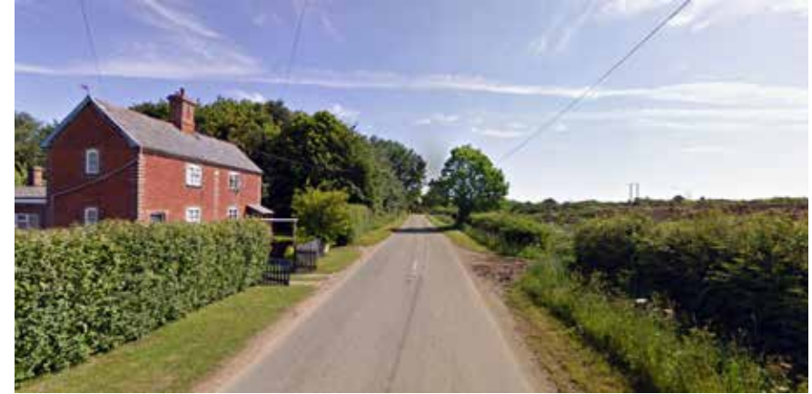
Figure 122: A pair of semi-detached cottages with hedgerows along Old Bury Road.
