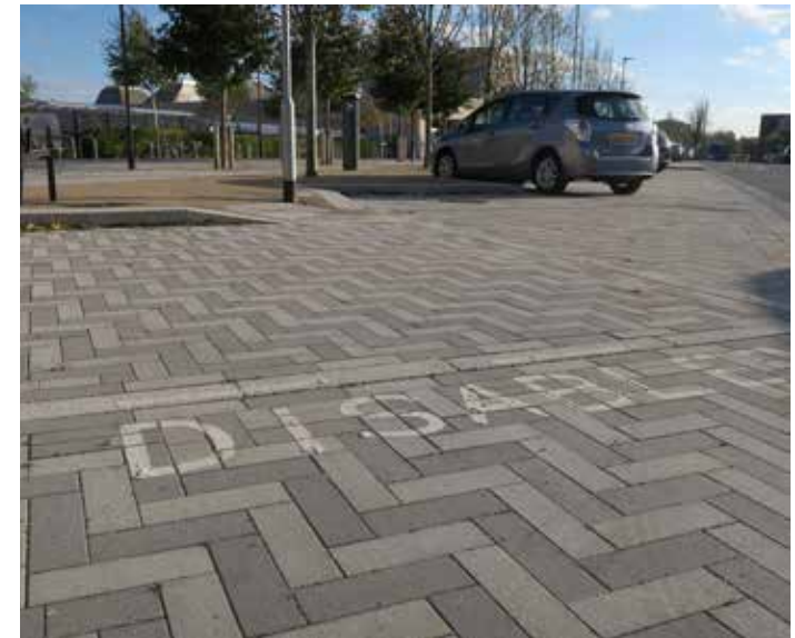
Figure 61: Disabled parking bay in Cambridge with ramp for easy wheelchair access.
