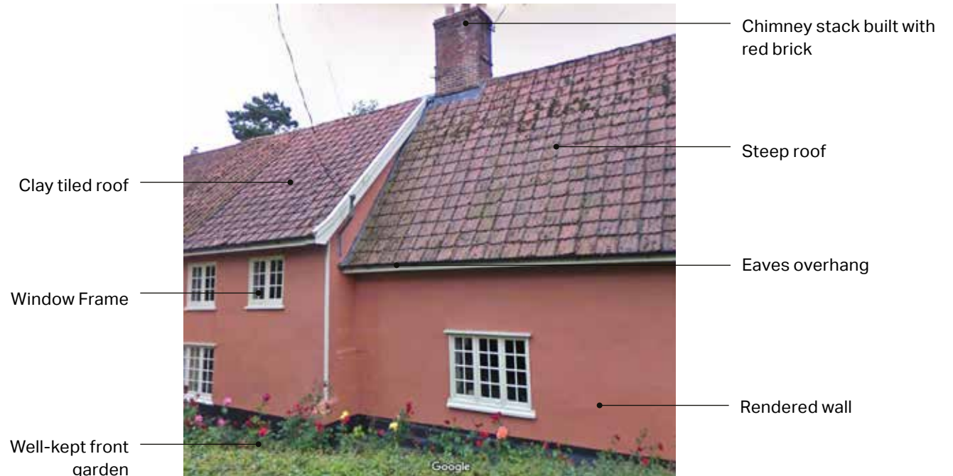
Figure 137: A detached residential house on Rectory Road.
