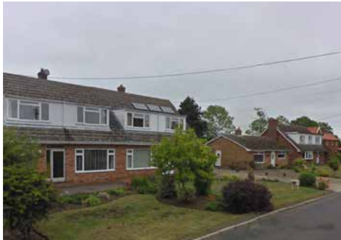
Figure 106: Two-storey semi-detached house On Crown Green, Burston.
