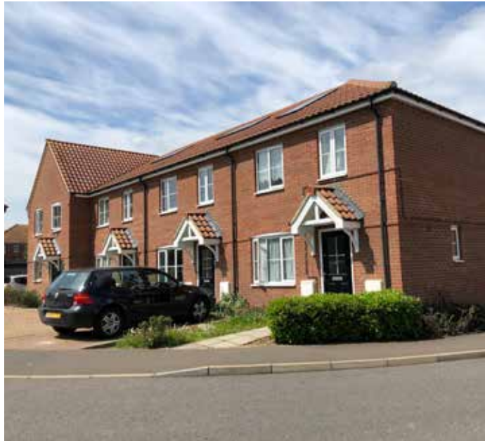
Figure 58: On-plot side parking on Spencer Crescent, Diss.
