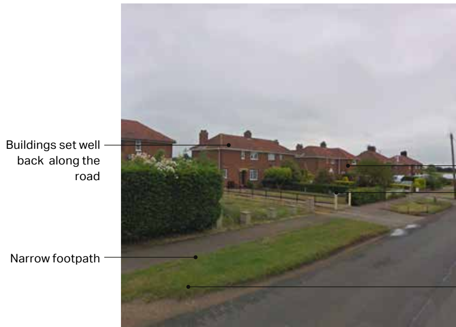
Figure 111: Boundary treatment on Station Road, Burston.
