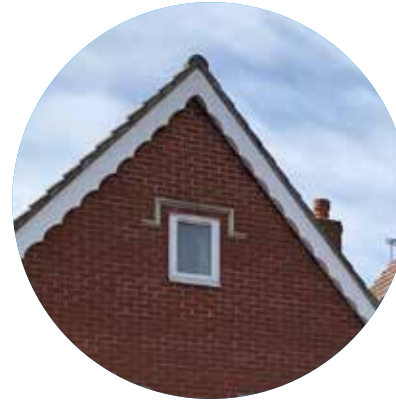
Decorative bargeboard gable
