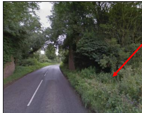
Road and embankment (channel shown by arrow). Photograph from Google Streetview
