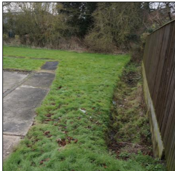
Upstream extent of DRAIN channel, looking downstream
