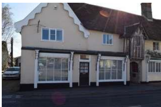
Traditional shop front windows
