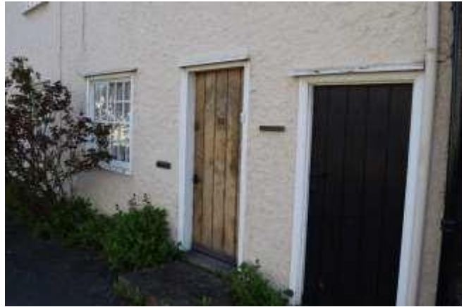
Timber 'cottage' style doors
