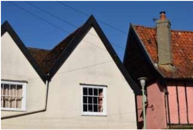
Black bargeboards, fascias and soffits
