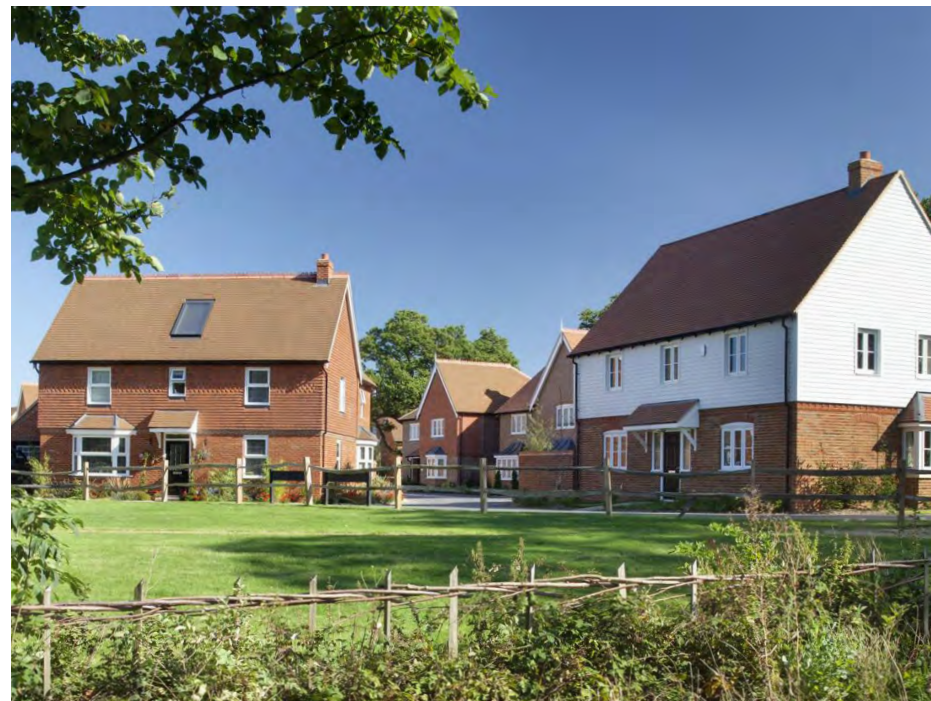
A new development with its own distinct character, which also integrates with its surroundings
