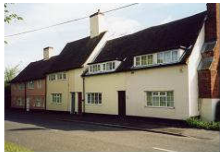
Smooth render, soft colours, dark plinths, vertical boarded doors, varied roof formations and building shapes
