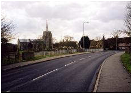
River bridge: ugly balustrading and wall, lighting, and pavings
