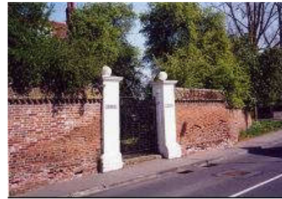
Piers and cappings are a strong village feature
