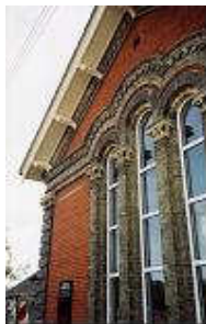
Contrasting bricks, formal architectural details, arches and overhanging roof giving contrast of light and shade
