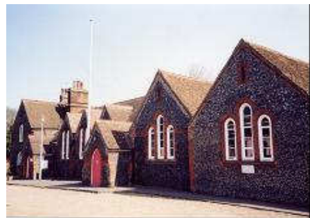
Flint, brick arches, varied frontages and variety of roof pitches
