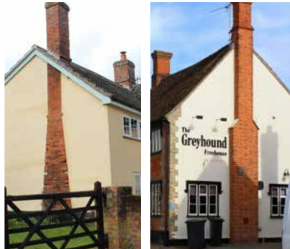
Figure 58: Brick chimney on pitched roof
