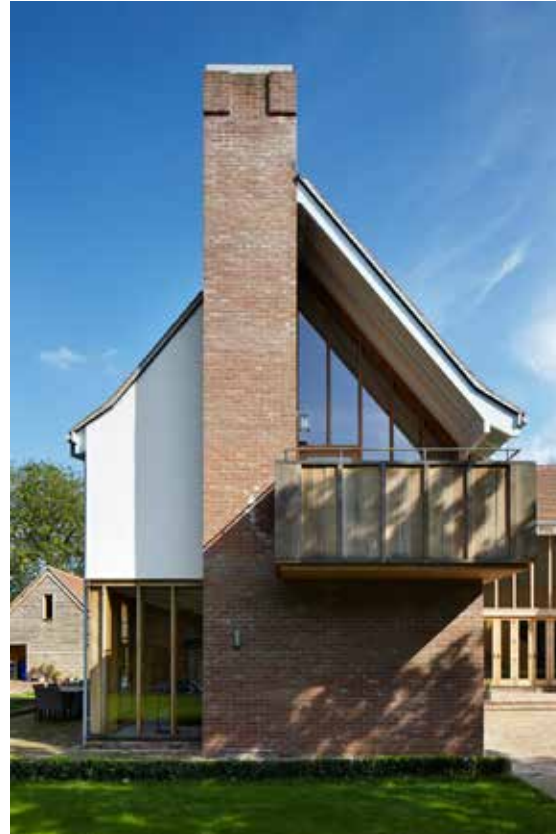
Example of contemporary architecture in West Stow, Bury St Edmunds. The image shows use of traditional features and materials in a contemporary design, such as a red brick chimney, the use of white render and red bricks and timber in the facade. Photo courtesy of Jack Hobhouse. Architects: Project Orange. Source: http://www.projectorange.com
