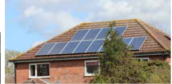
Figure 60: Solar panel on shallow hipped roof
