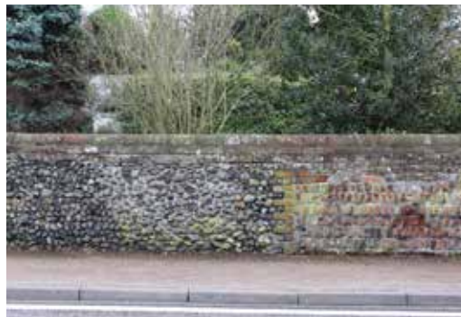
Figure 35: Traditional boundary treatment in Suffolk
