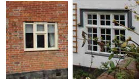
Figure 62: Casement window details
