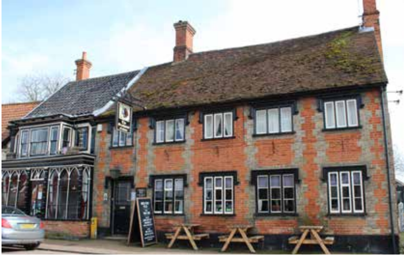
Figure 48: The Greyhound public house with brick facade and traditional windows
