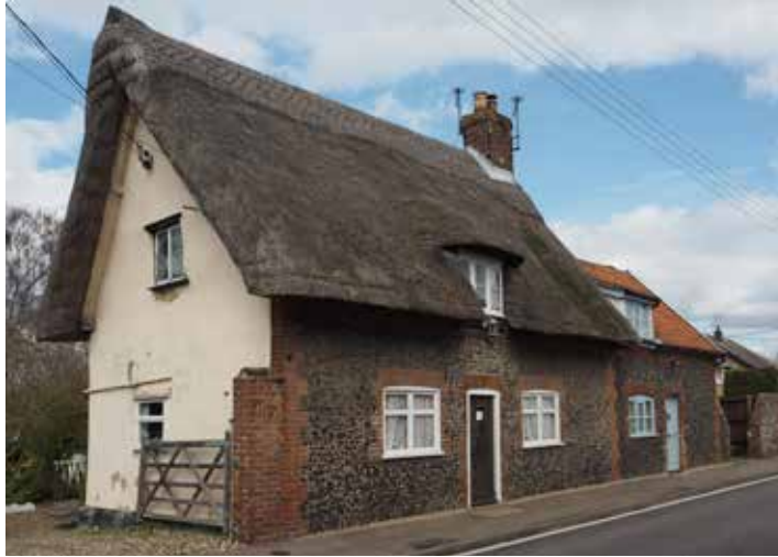
Figure 50: Typical architectural building with thatched roof, flint and red brick facade and ornamental windows
