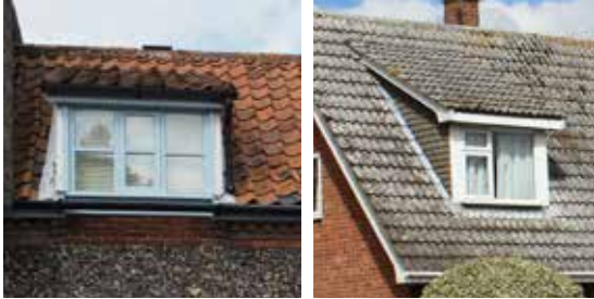
Figure 55: Shed Dormer Window
