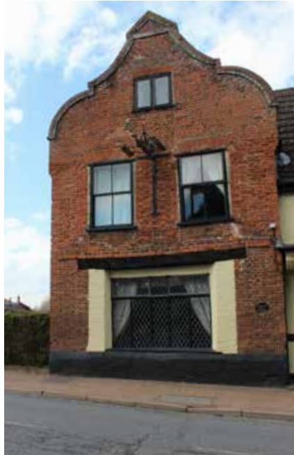
Figure 46: Hamblyn House with red brick facade and timber structure
