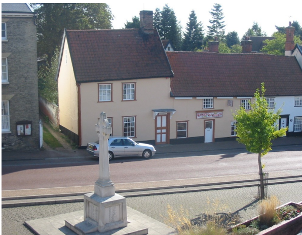
Tudor House and Tudor Cottage, Market Place
