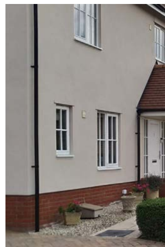
Figure 12: Low skirting on The White Horse and similarly on new developments
