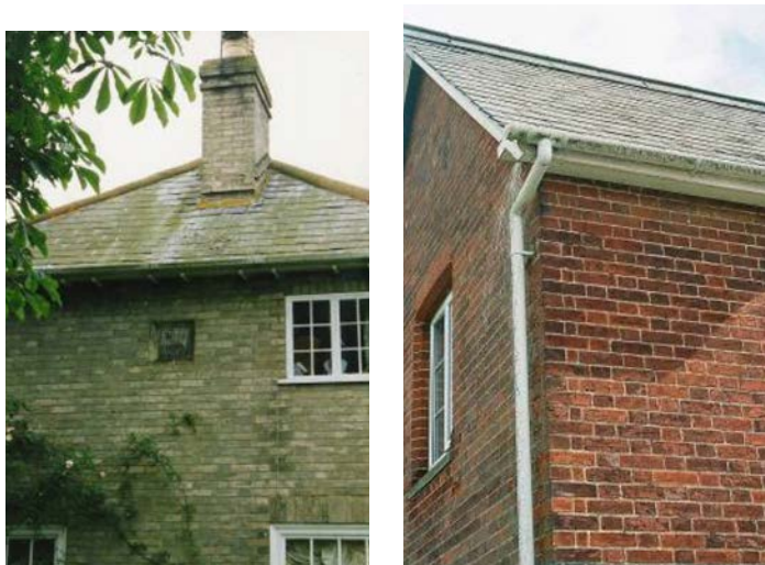
Figure 10: Traditional facade finishes taken from Beyton examples
