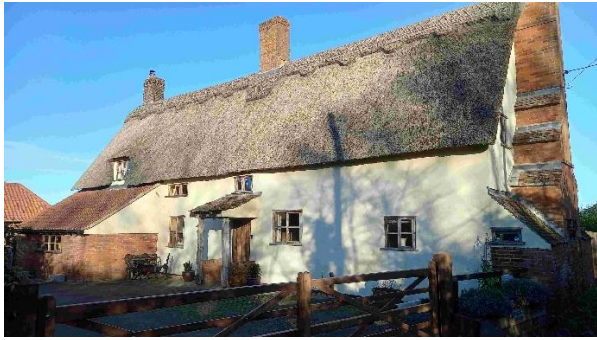
1 – Hill Top Farmhouse (Outbuilding 2 was not accessible)
