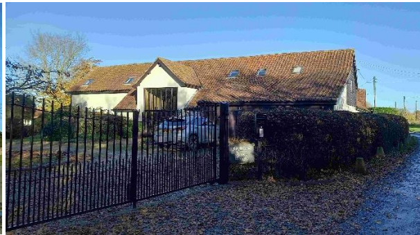
4b – The barn in the curtilage of Stone Farm House
