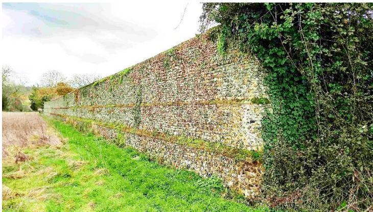
38: The flint walls to the north-west of Church Lane
