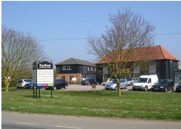
Figure 48: Contemporary commercial buildings with traditional roof and exterior designs.
