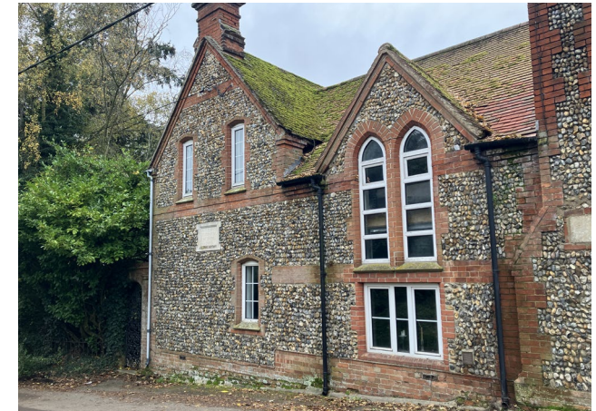
Figure 14: The National School with flint walls and red-brick detailing. An example of a valuable non-designated heritage asset within the village.
