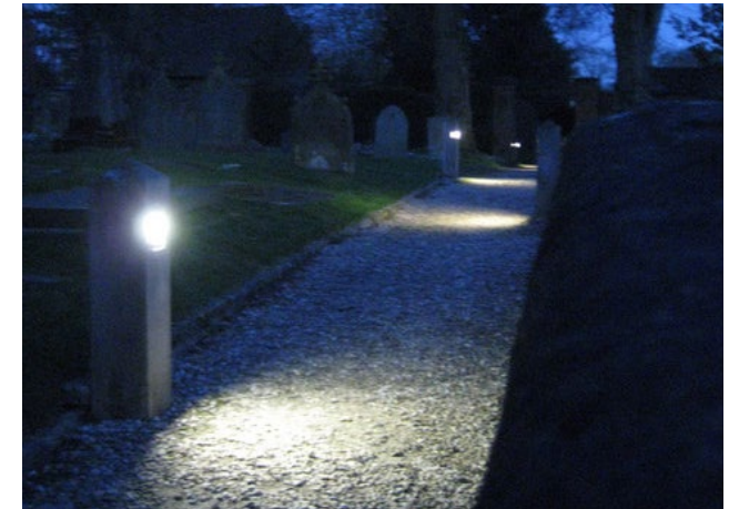
Figure 40: Example of a low-level lighting solution at Lapworth churchyard (photo: Robin Stott).
