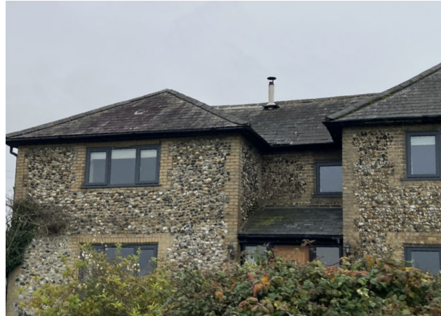
Figure 36: High quality material choice used for a retrofit of windows.
