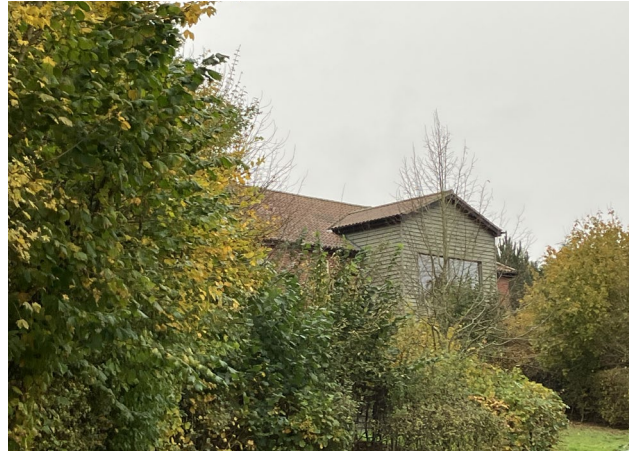
Figure 25: Landscaping used to screen Baylham Care Centre from Upper Street, integrating the development within the surrounding landscape.
