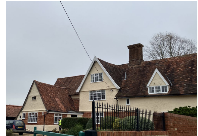
Figure 15: Stone Farm, a Grade II listed 16th century farm house with a typically historic farmstead layout set along the Circular Road.
