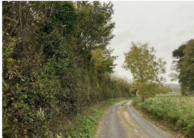
Figure 30: Dense bounding hedgrows providing side friction, alongside a loose surface and narrow, meandering character. This enables traffic calming while underpinning the rural feel of peripheral areas of the village.
