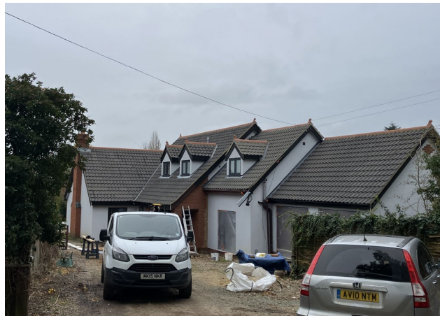
Figure 38: An additional example of a contemporary home under construction with contemporary iterations of traditional features, including colour render, narrow gable dormers and glazed slate pantiles.
