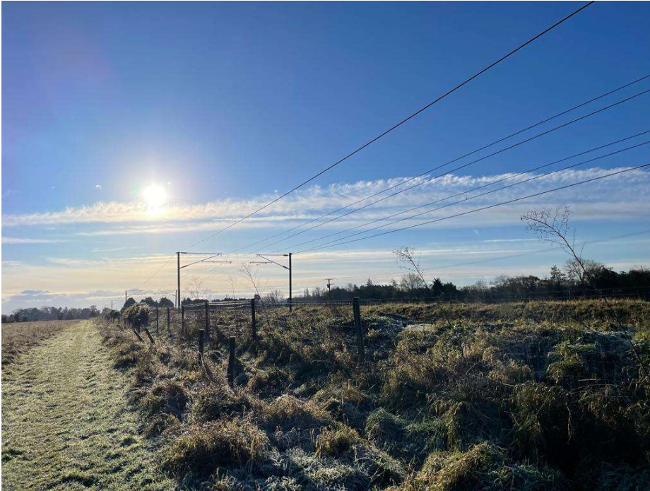
Railway track running through east of Baylham, looking south.
