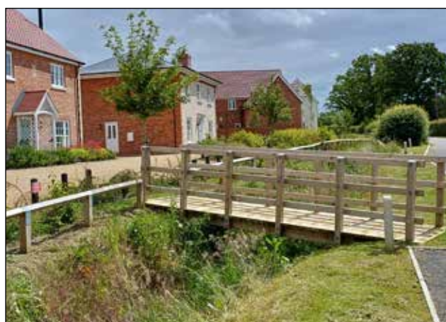
Figure 61: Example of a swale along The Broadway integrated into a new development within Badwell Ash village.
