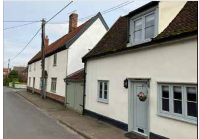
Figure 06: White render cottages with wooden casement windows and brick or painted stone base plinths.
