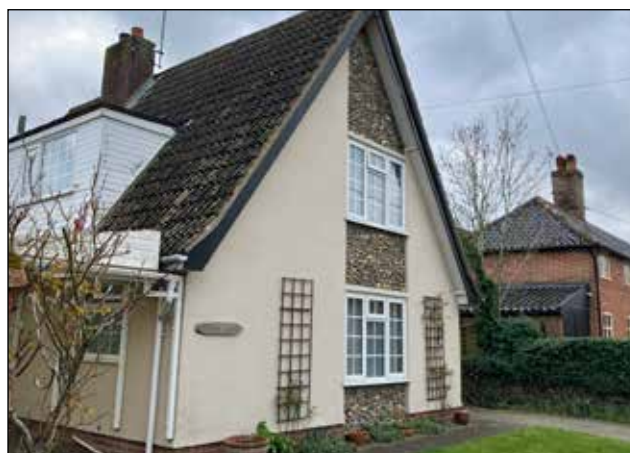
Figure 55: Example of appropriate materiality on 20th century dwelling.
