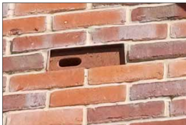
Figure 65: Example of a swift brick installed on a dwelling in the Parish.
