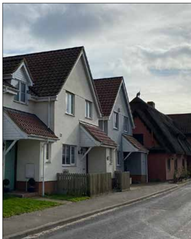
Figure 48: Recent infill development retaining the existing building line along The Street.
