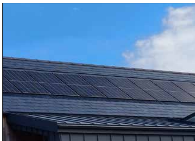
Figure 57: Example of discreet solar panels that sit flush within the roof tiles.
