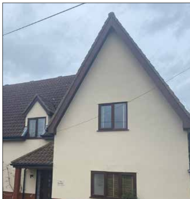
Figure 31: Pitched dormer and gable front with pronounced roof pitch.
