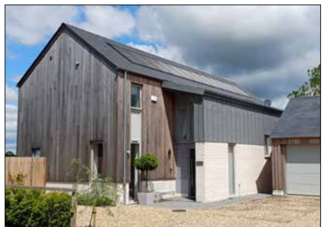
Figure 08: Contemporary architecture in Long Thurlow with larch timber cladding and slate roof.
