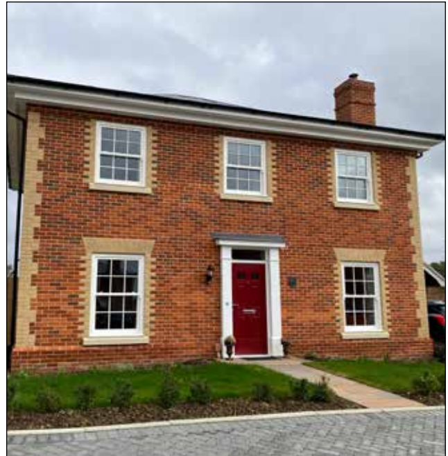
Figure 34: Red brick facade with light brick detailing.
