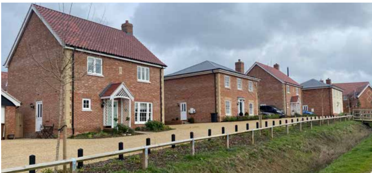
Figure 44: Recent dwellings in Badwell Ash village fronting onto landscaping integrated into swale.
