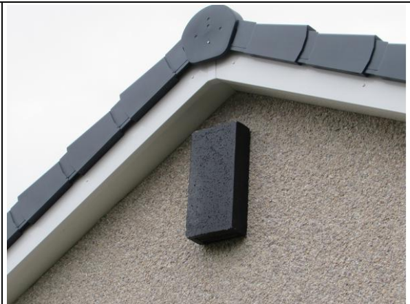
Example of a bat box attached to a new building
