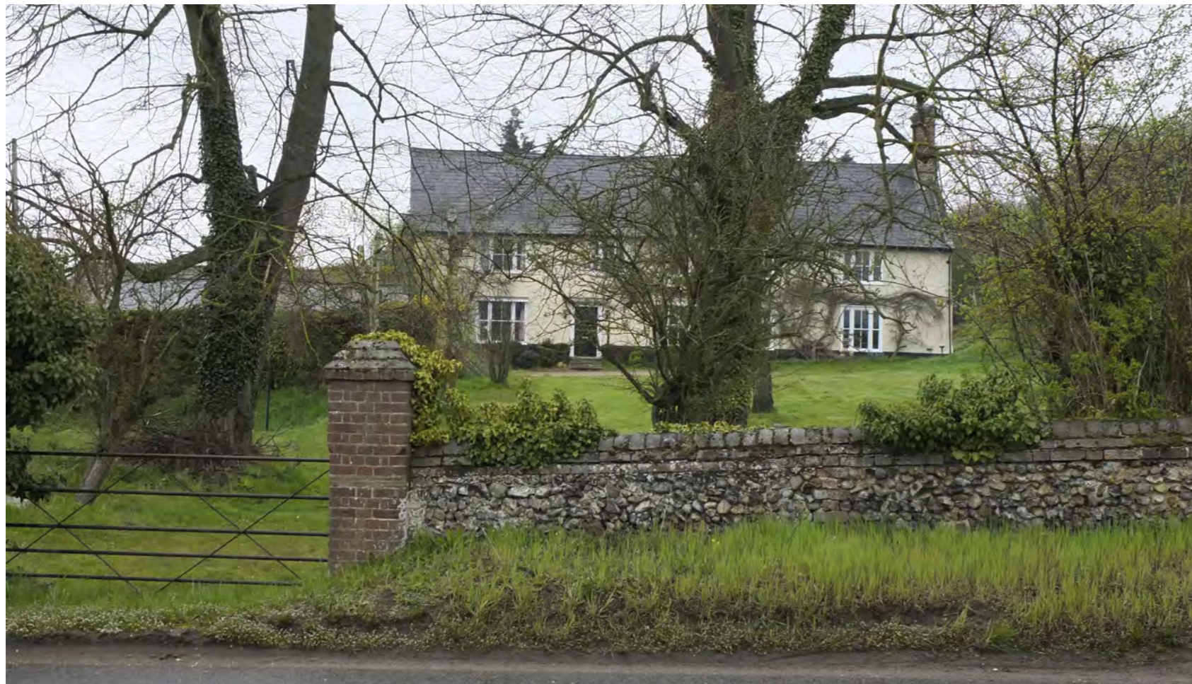
Ashes Farm listed building
