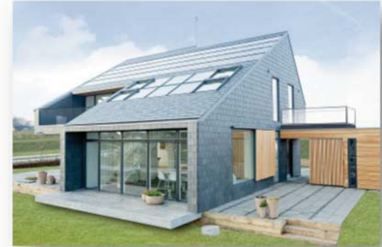
Images - Above: New housing can take full advantage of solar power with integrated panels on southern faces. Aarhus, Denmark house for life: www.activehouse.com and www.aart.dk .
