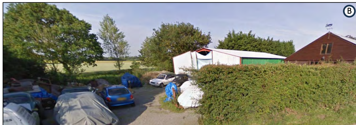
figure 102: Buildings east of Capel Station Garage
