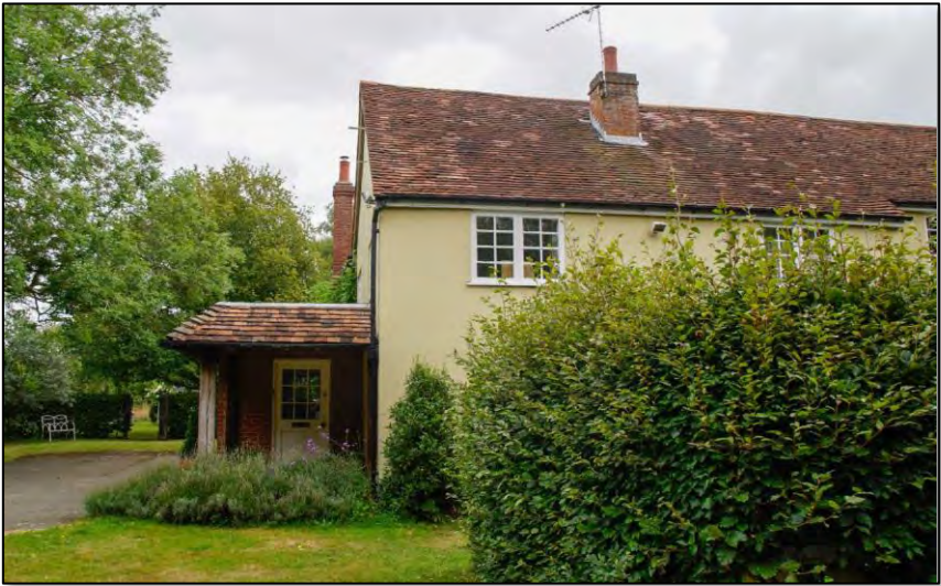
figures 187: Church Farm non-designated heritage asset
