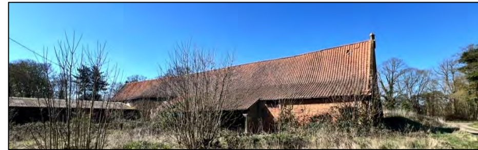
figure 136: Bentley Hall Barn [Grade I listed building]
