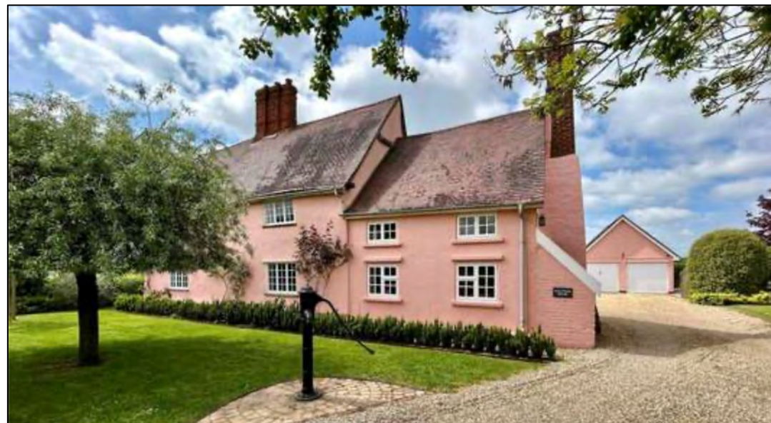
figure 98: Maltings House [front]
