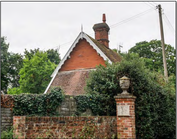
figures 186: Hope Lodge: non-designated heritage asset of Local Significance
