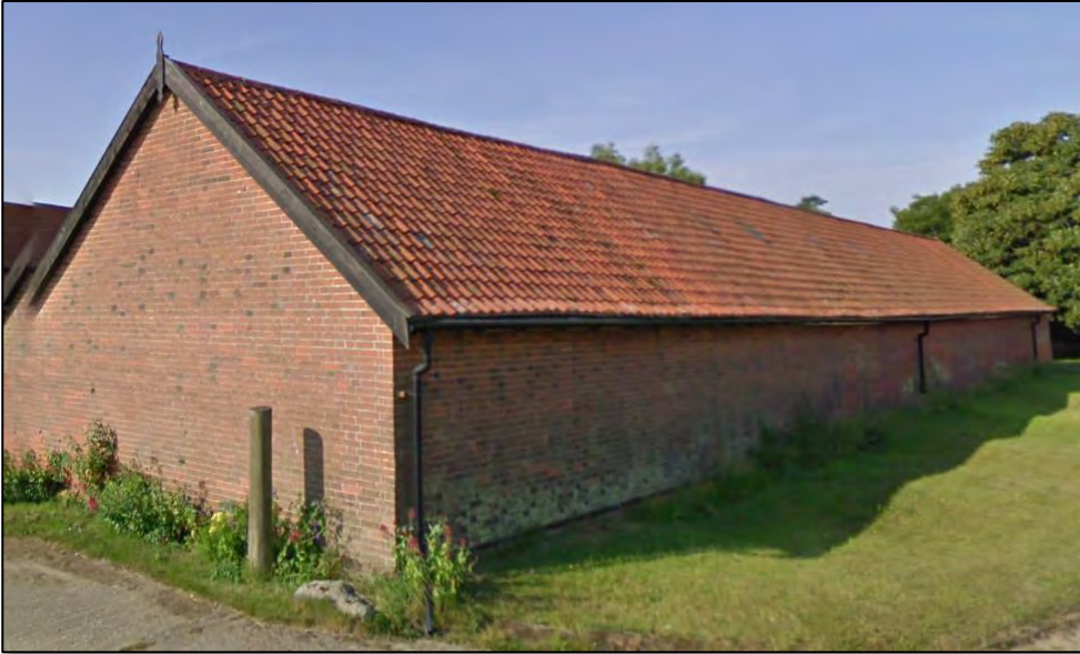
figure 79: Brick barn to road frontage - Pond Hall
