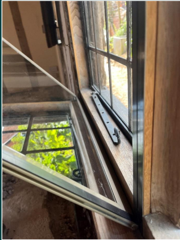
Good example – This secondary glazing to a timber framed window with metal casements is held in place by magnetic tape
