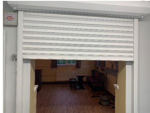
Newly installed Fire Shutter
