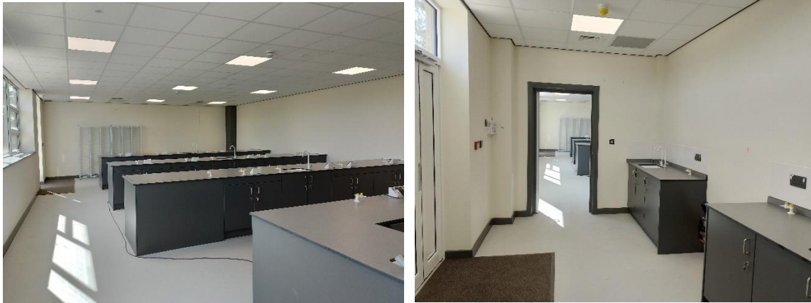
A view of one of the science labs and the connecting prep room.
