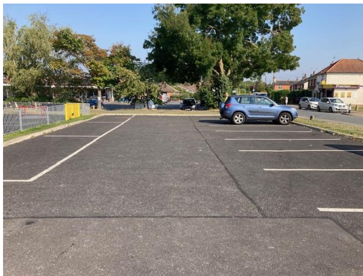
The completed extension to the car park
