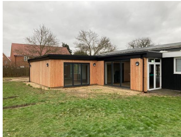
The new extension as viewed from the rear of the Village Hall
