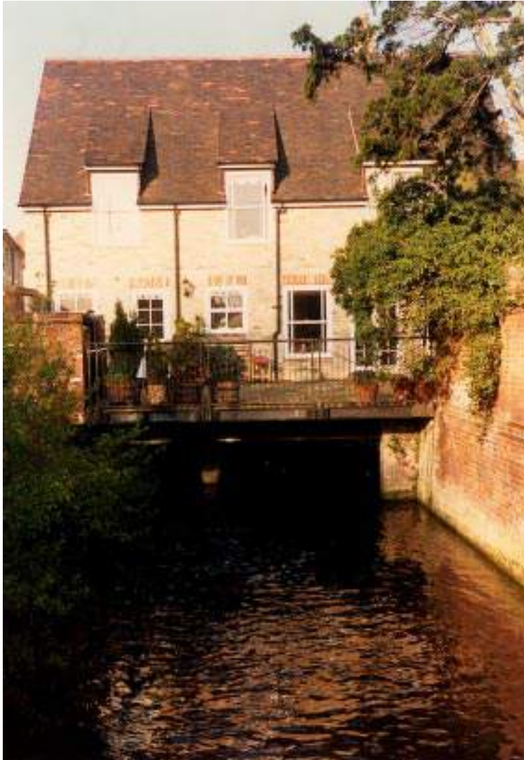
View from bridge over Mill Lade.
