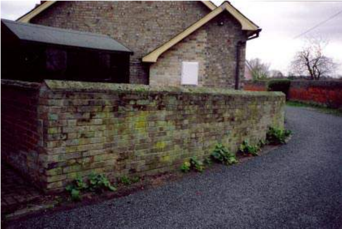
Suffolk white brick wall approximately. 7 metres long, between No. 10 and The Almshouses (Nos. 12-16).
