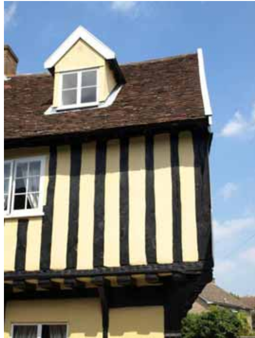
Exposed Timber Frame, Plaintile
