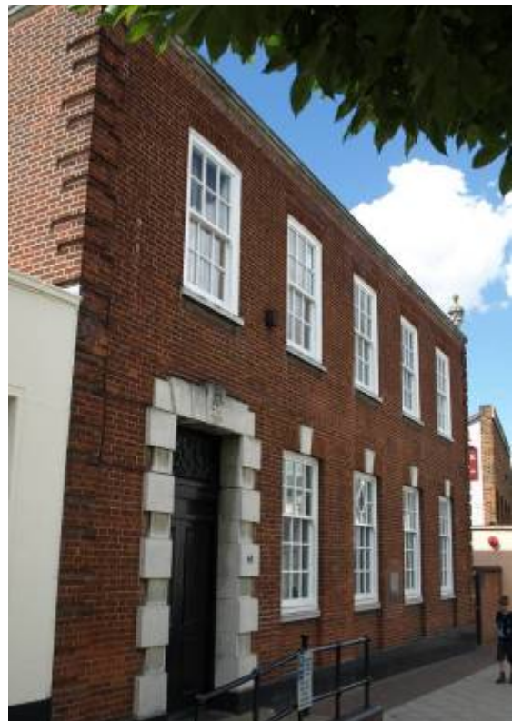
Former Post Office
