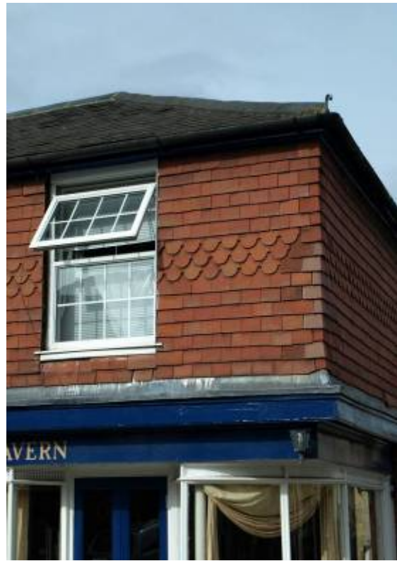
Tile-hanging and Slate
