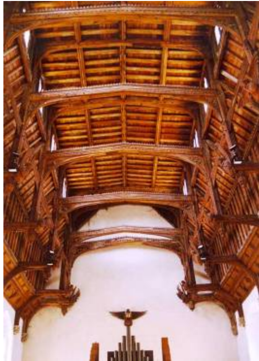
Hammerbeam Roof
