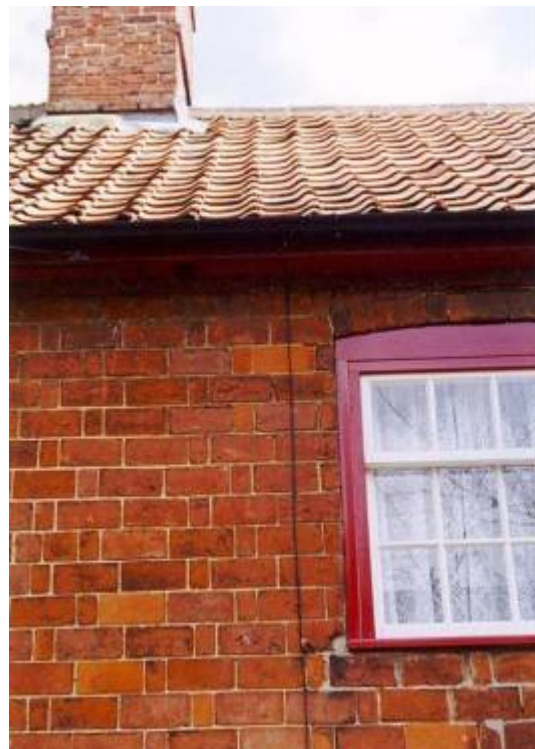
Rat-trap Bond and Pantile
