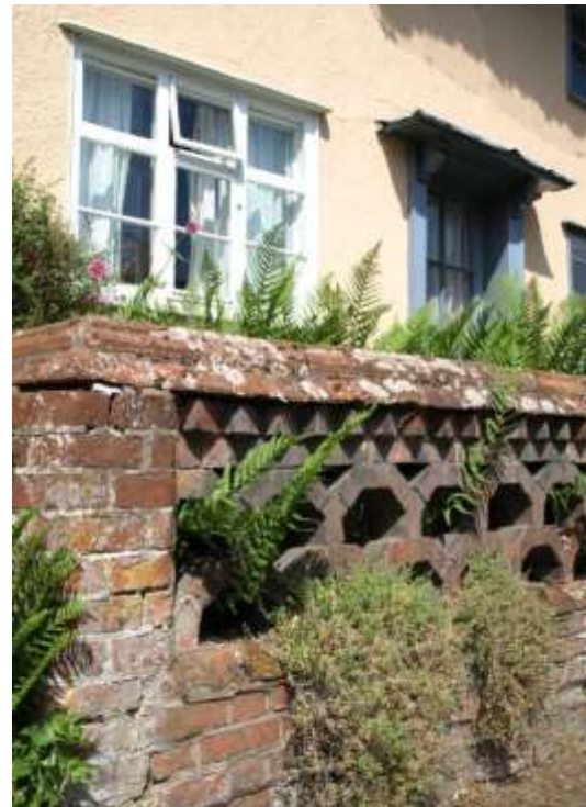
Banham Brick Walls
