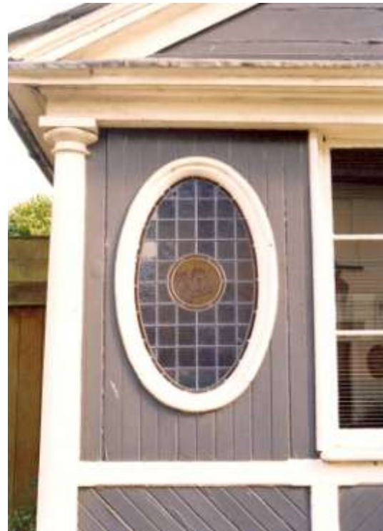
'Classical' Timber Boarding
