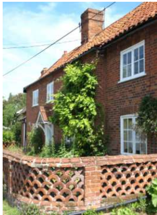
Banham Brick Wall, Cross Street
